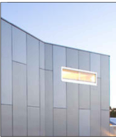
FRAMED SHEET CLADDING
