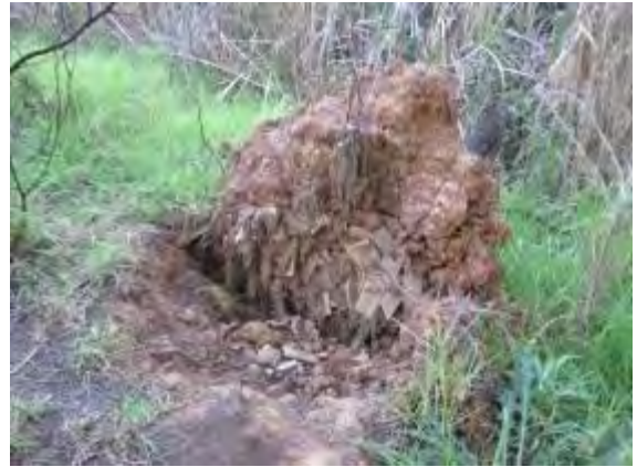
Plate 10. Exposed fill material in disturbed area
