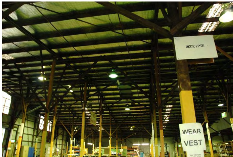
Figure 19: Interior of Building 79, showing original timber post and beam construction
