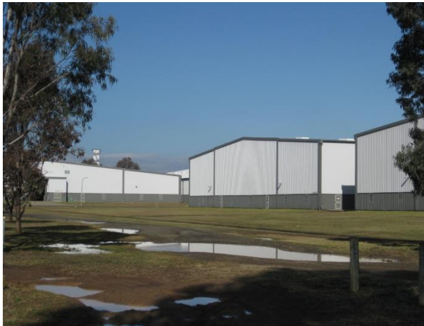
PICTURE 7 – EXISTING WAREHOUSE BUILDINGS
