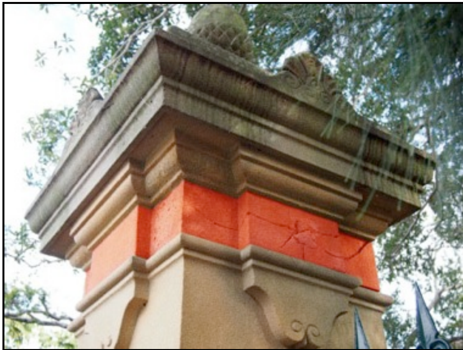
Figure 10 Install hairline indent to cap as shown in red prior to reinstatement. (Photo: Jasper Swann, 2013)
