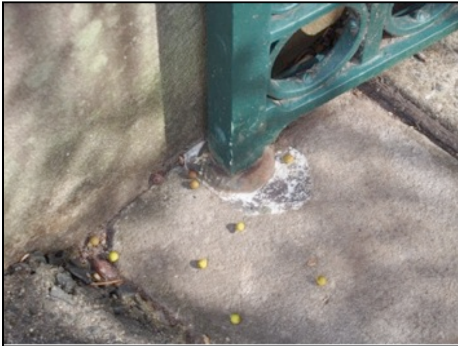
Figure 4 Iron ferrule at pivot of gate. Remove and retain in storage for future use. (Photo: Jasper Swann, 2013)
