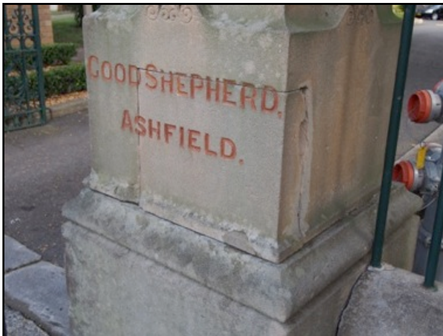
Figure 5 Existing indent in Pier 2. Care required when dismantling. (Photo: Jasper Swann, 2013)
