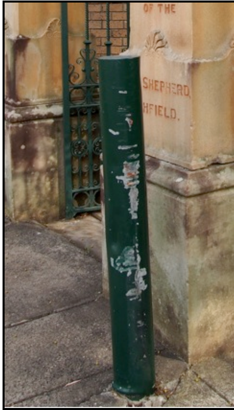
Figure 8 Existing steel bollards (2 Off) to be removed and temporarily re-instated to protect exposed ends of railing base during construction. (Photo: Jasper Swann, 2013)
