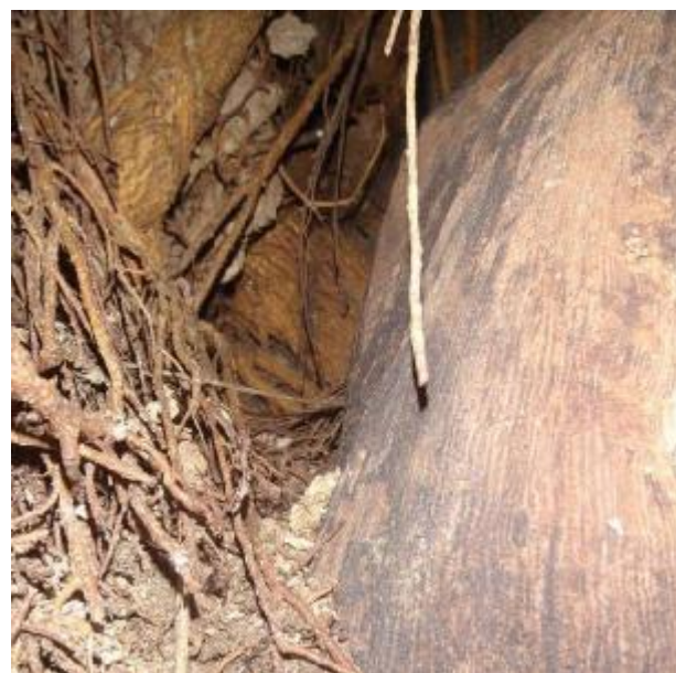
Image 11: Roots clearly visible inside cavity
