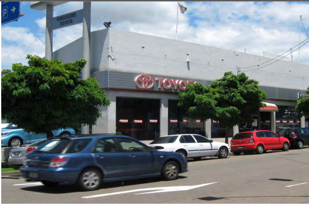
PHOTO P3 No. 23 Office Building
