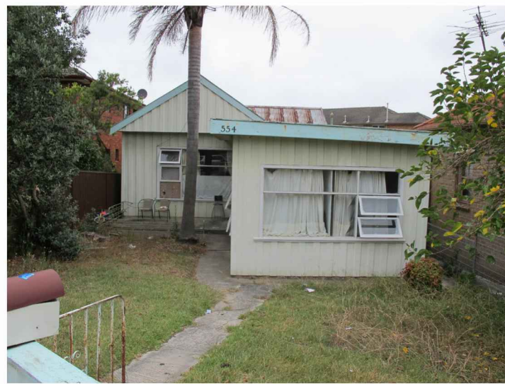
554 RAILWAY PDE VIEW FROM RAILWAY PDE
