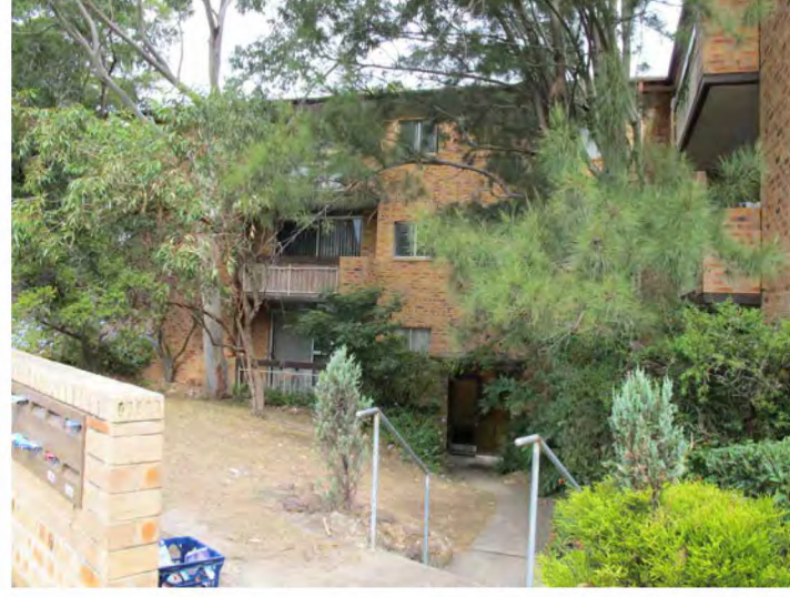
516-520 RAILWAY PDE VIEW FROM RAILWAY PDE 4ST(3R)
