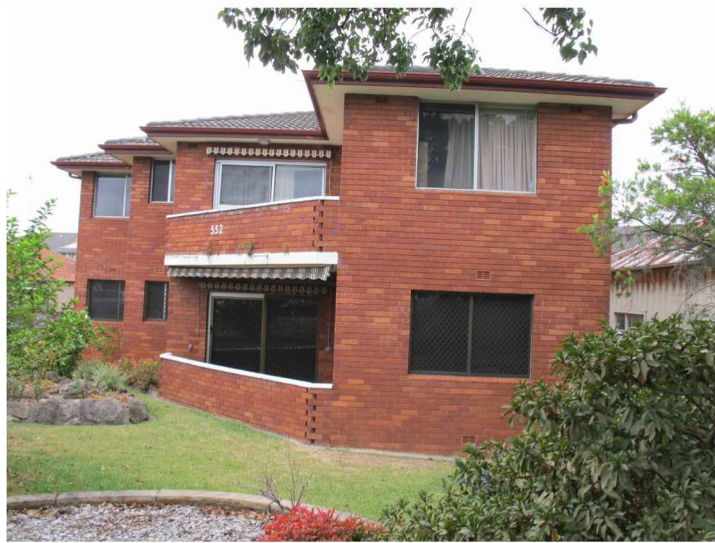
552 RAILWAY PDE VIEW FROM RAILWAY PDE
