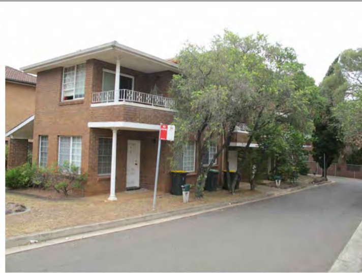
3 BELLEVUE LN - VIEW FROM CORNER OF BELLEVUE LN & WOIDS AVE 2ST/ 3ST , 2 LEVEL DWELLING
