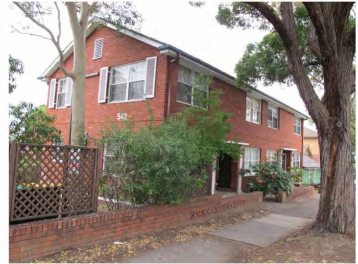
542 RAILWAY PDE VIEW FROM ST GEORGES PDE 2ST, 2 LEVEL DWELLING
