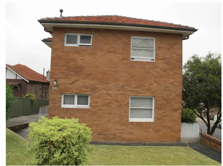
558 RAILWAY PDE VIEW FROM RAILWAY PDE
