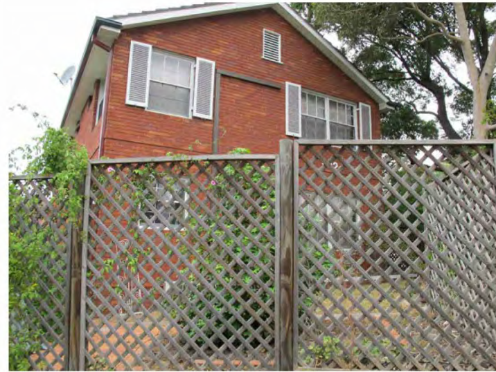
542 RAILWAY PDE VIEW FROM RAILWAY PDE 2ST, 2 LEVEL DWELLING
