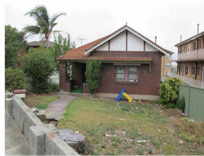
556 RAILWAY PDE VIEW FROM RAILWAY PDE
