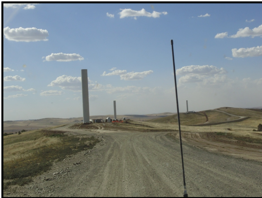
Figure 5.1: Typical unsealed access road within a wind farm site
