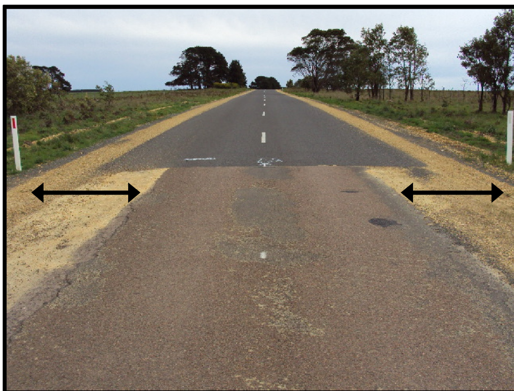
Figure 5.2: Typical unsealed increase in width of (public) road
