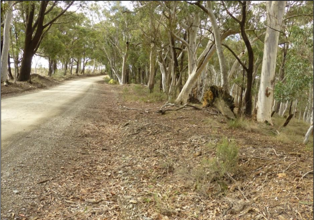
Grade 2: LHS - Would require minor clearing and levelling, straight section of road.
