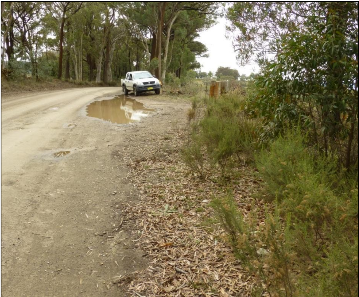
Grade 1: LHS - Located at a driveway. Cleared section exists, some clearance may be required.
