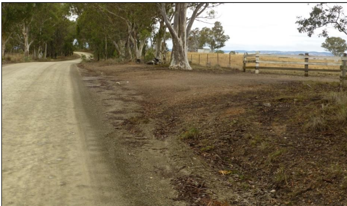
Grade 1: LHS - Located at a driveway. Straight section of road.
