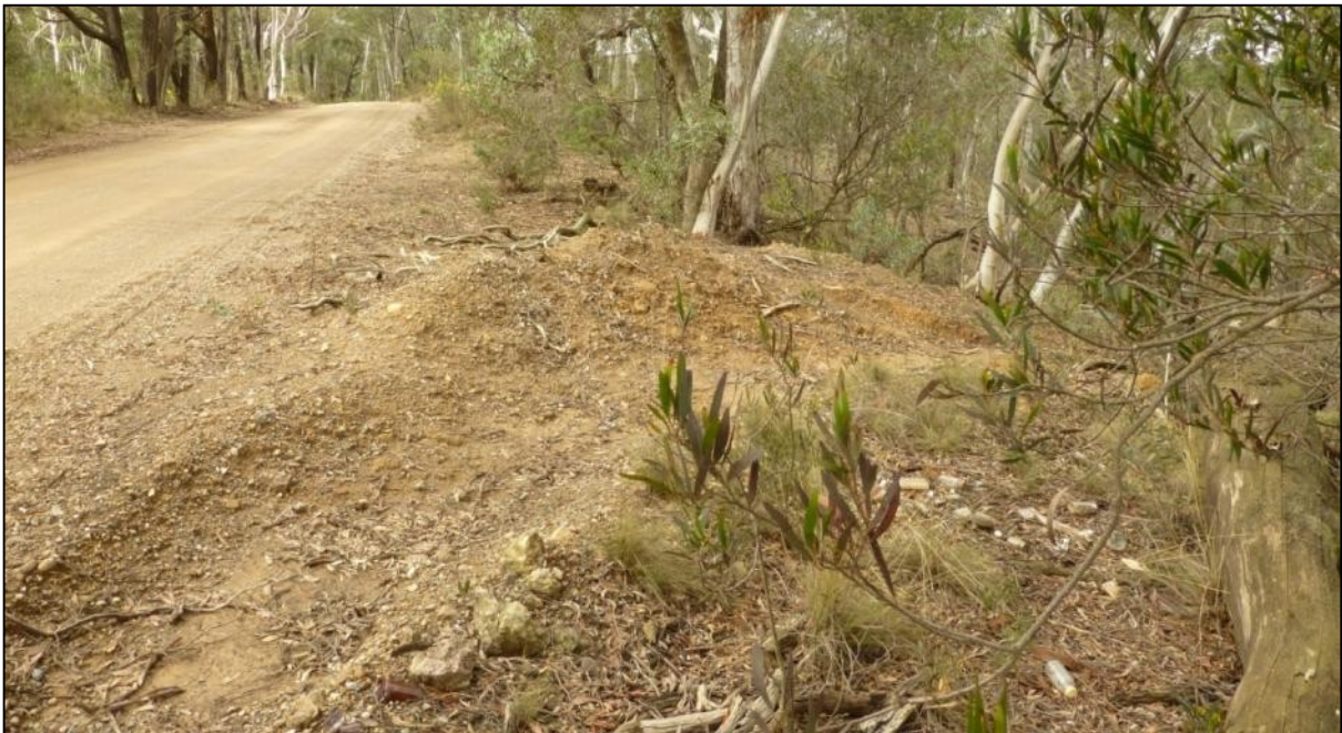
Grade 3: LHS - Clearance and levelling required, straight section of road.
