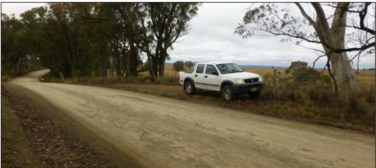
Grade 1: LHS - Minor clearing required, large area and straight section of road.
