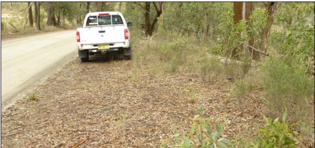
Grade 3: RHS - Clearance and levelling required, on straight section of road.
