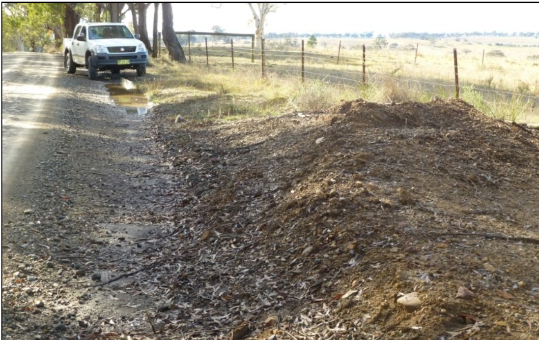
Grade 3: LHS - Minor clearing required. Some levelling required. Not as wide as other locations.
