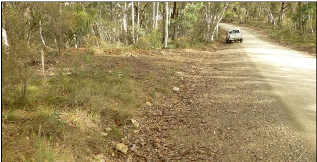
Grade 1: LHS - Clearance and levelling required, on straight section of road.
