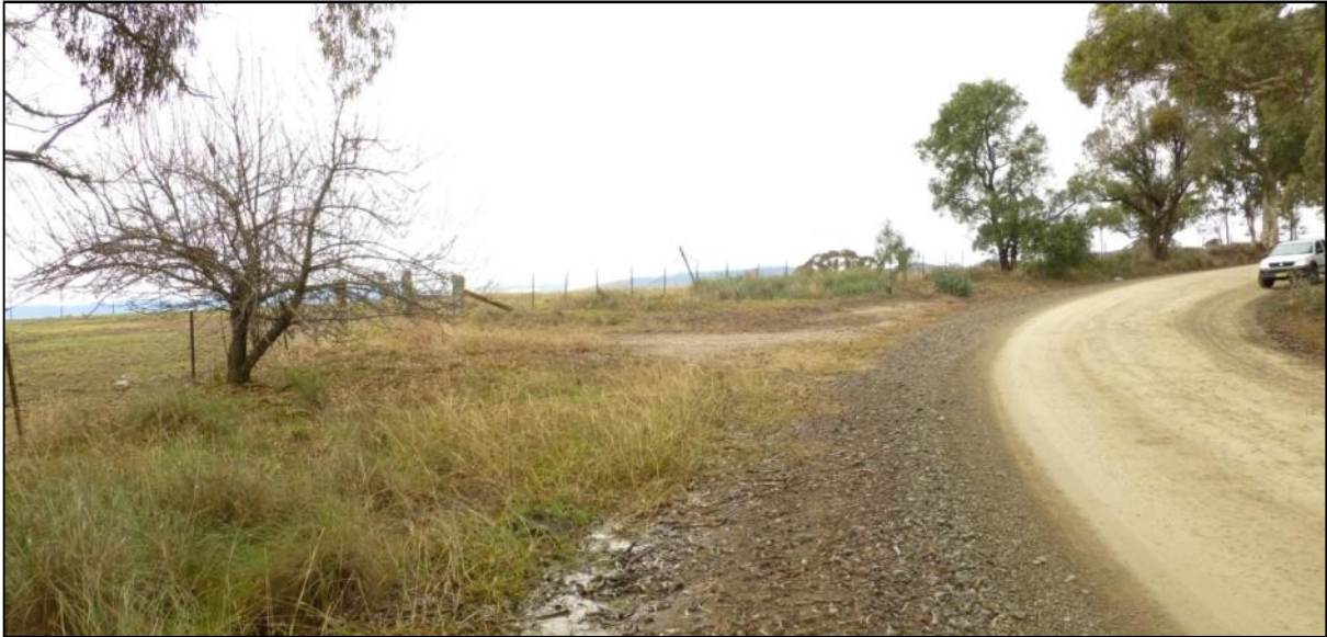
Grade 3: RHS - Located at a driveway. Minor clearing required, on a left bend.
