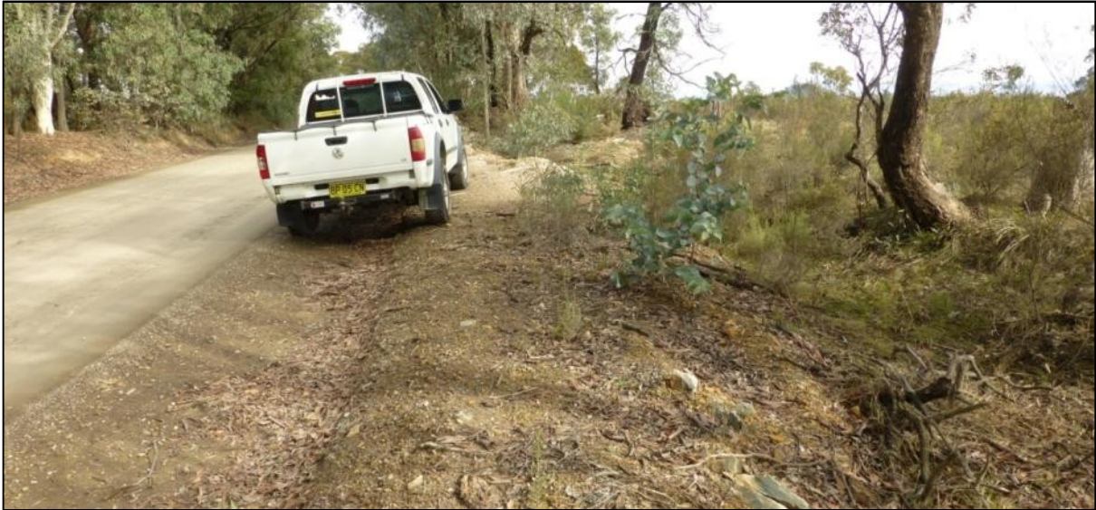
Grade 3: RHS - Some clearance and levelling required. On slight right bend
