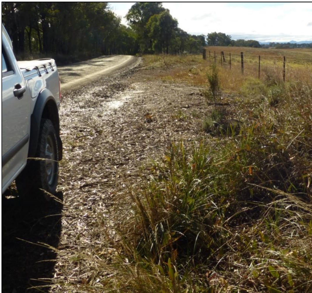
Grade 1: LHS - Straight section of road. Some levelling and clearing required.
