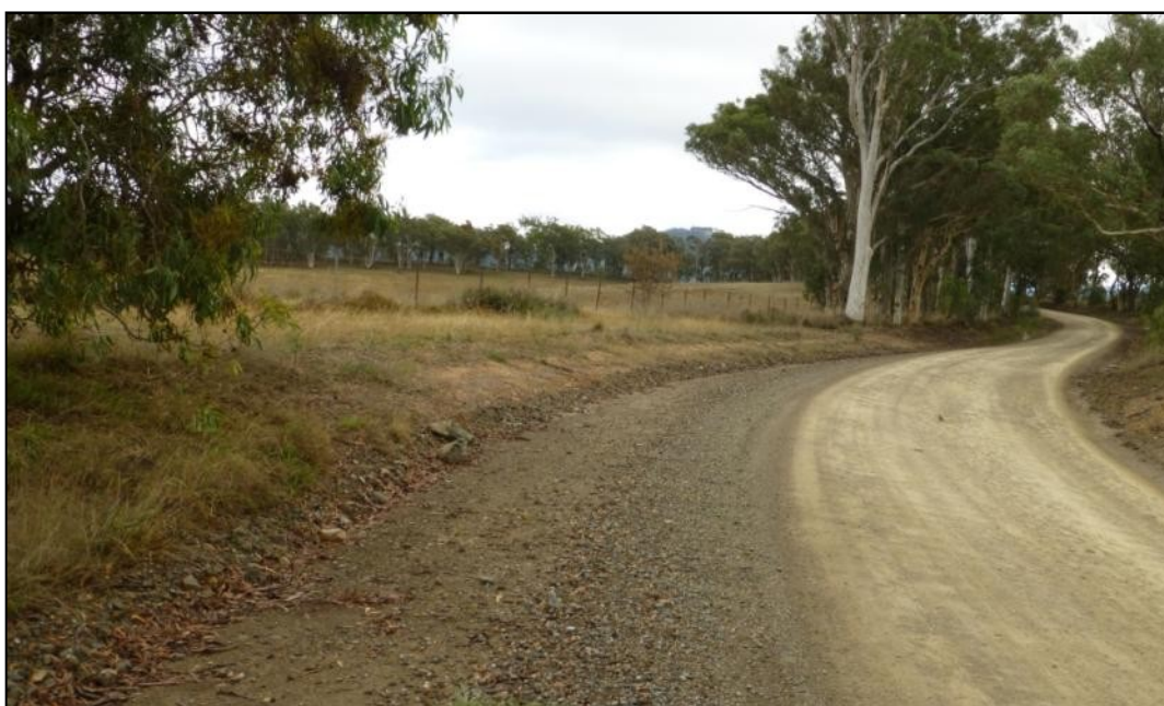
Grade 1: LHS - Large existing clearing, some levelling required.
