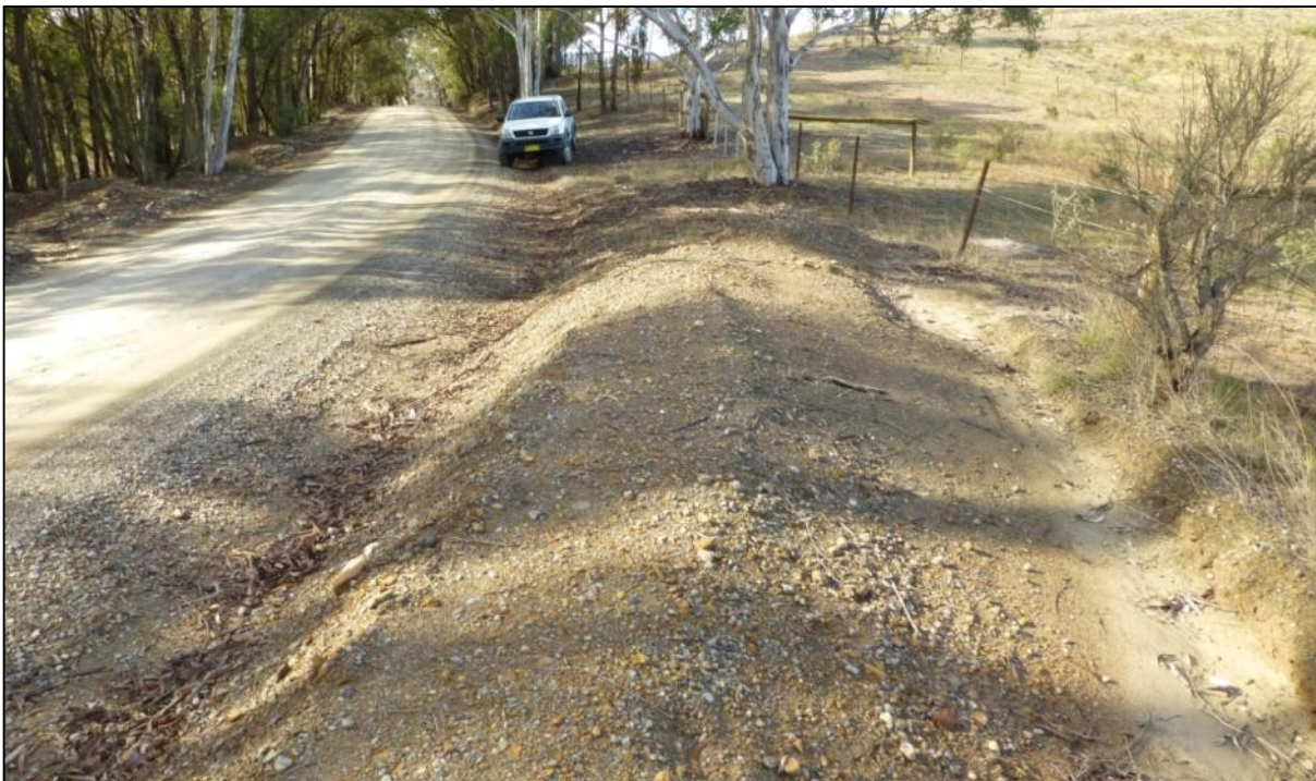
Grade 2: LHS - Some levelling required, minor clearing required. On a slight right bend.
