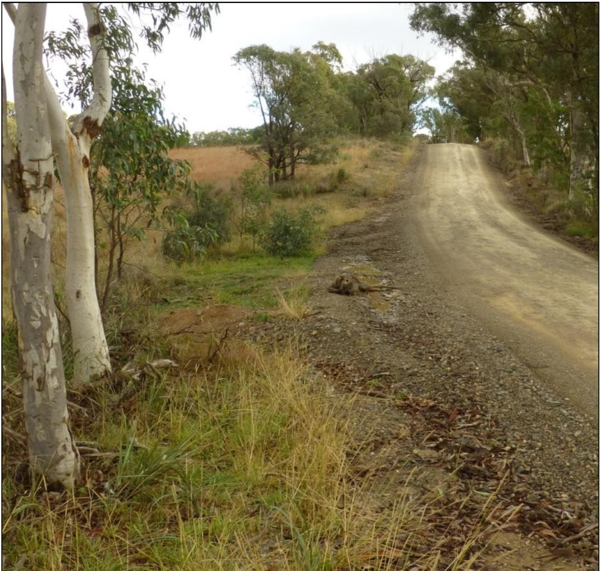
Grade 3: LHS - Some clearing required, located on a straight section of road, however the road is sloped at this location.
