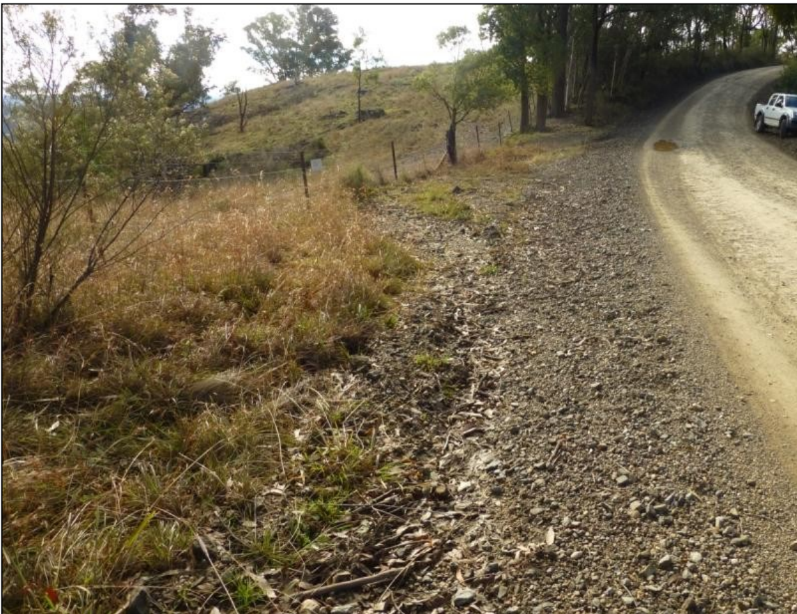
Grade 2. RHS - Low level of clearing and levelling (fill) required, on a slight right bend
