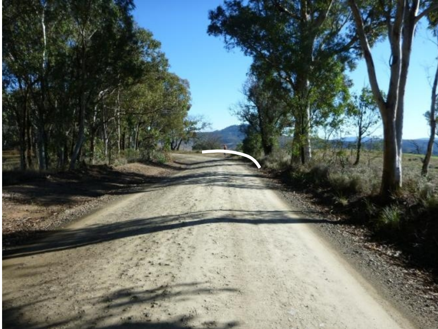
Plate 8 Location of Upgrade 3.5 ; looking 300°.
