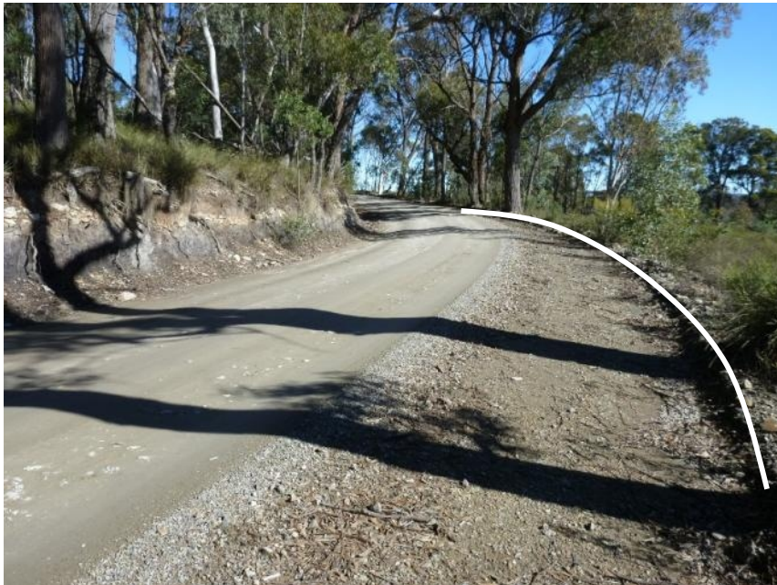
Plate 30 Location of Upgrade 3.16 ; looking 210°.
