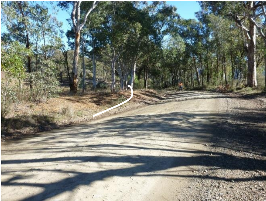
Plate 13 Location of Upgrade 3.9 ; looking 260°.
