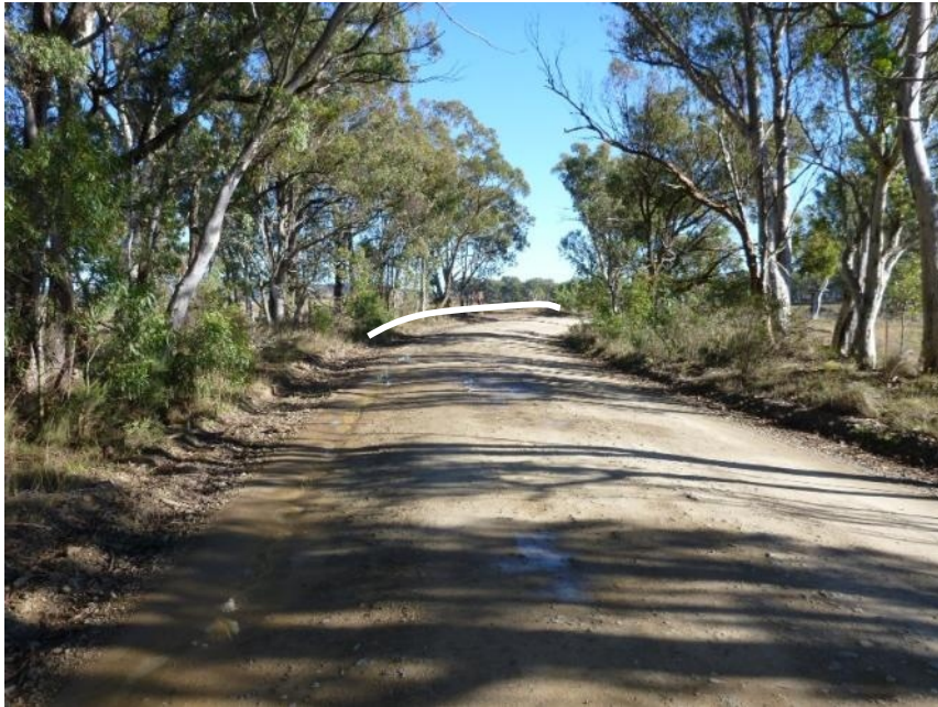
Plate 6 Location of Upgrade 3.4 ; looking 260°.
