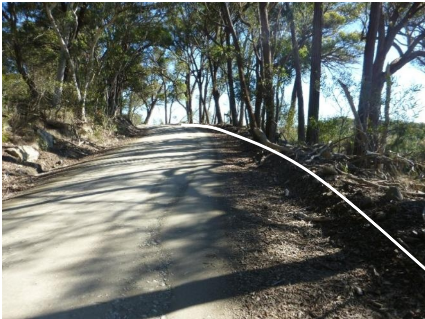
Plate 34 Location of Upgrade 3.18 ; looking 250°.
