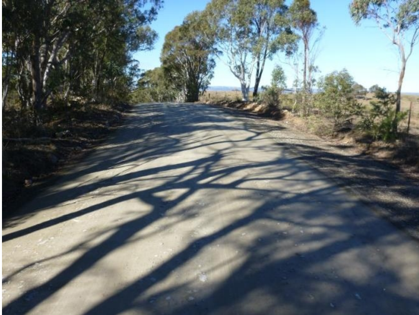
Plate 23 Location of Upgrade 3.12 ; looking 120°.
