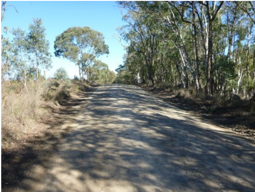
Plate 18 Location of Upgrade 3.10 ; looking 210°.
