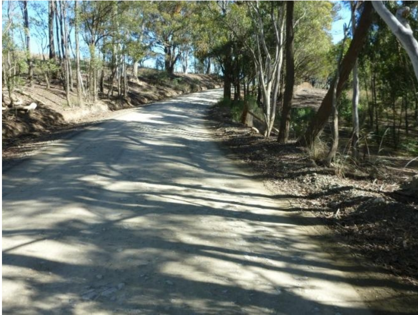
Plate 21 Location of Upgrade 3.11 ; looking 260°.
