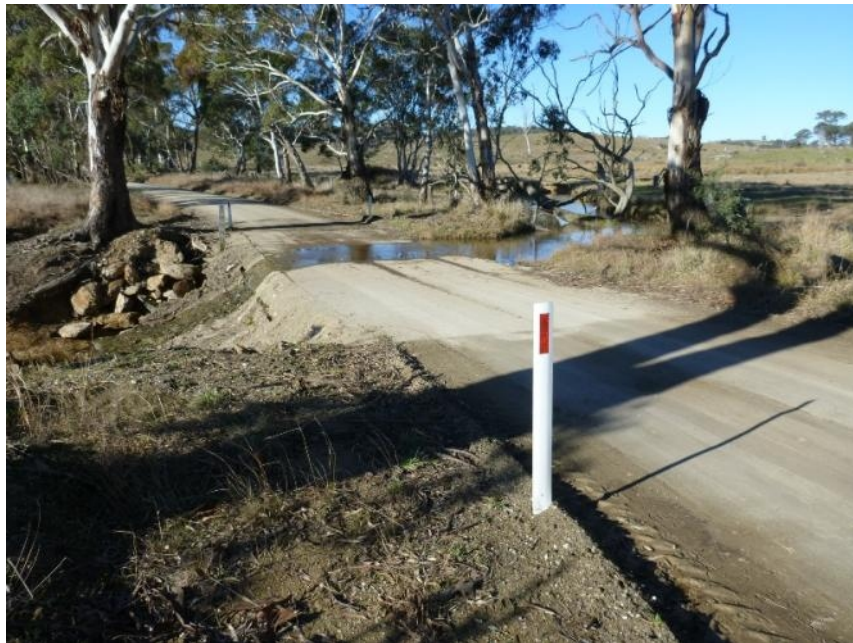
Plate 59 Location of Upgrade 3.30 ; looking 60°.
