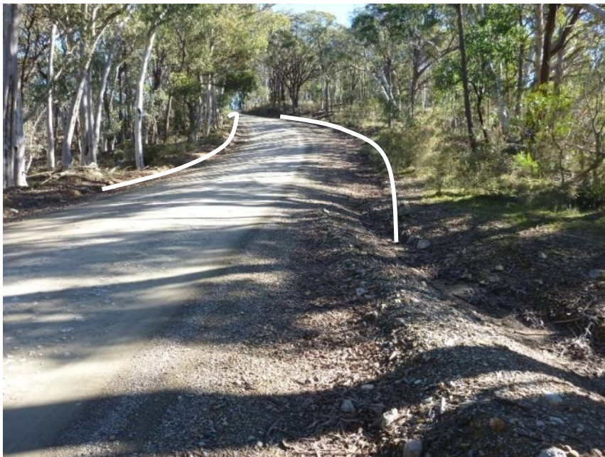
Plate 42 Location of Upgrade 3.22 ; looking 240°.
