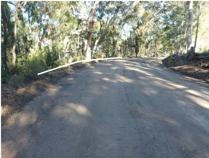
Plate 52 Location of Upgrade 3.26 ; looking 150°.
