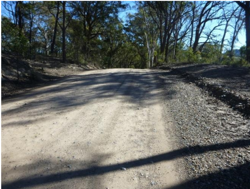
Plate 38 Location of Upgrade 3.21 ; looking east.
