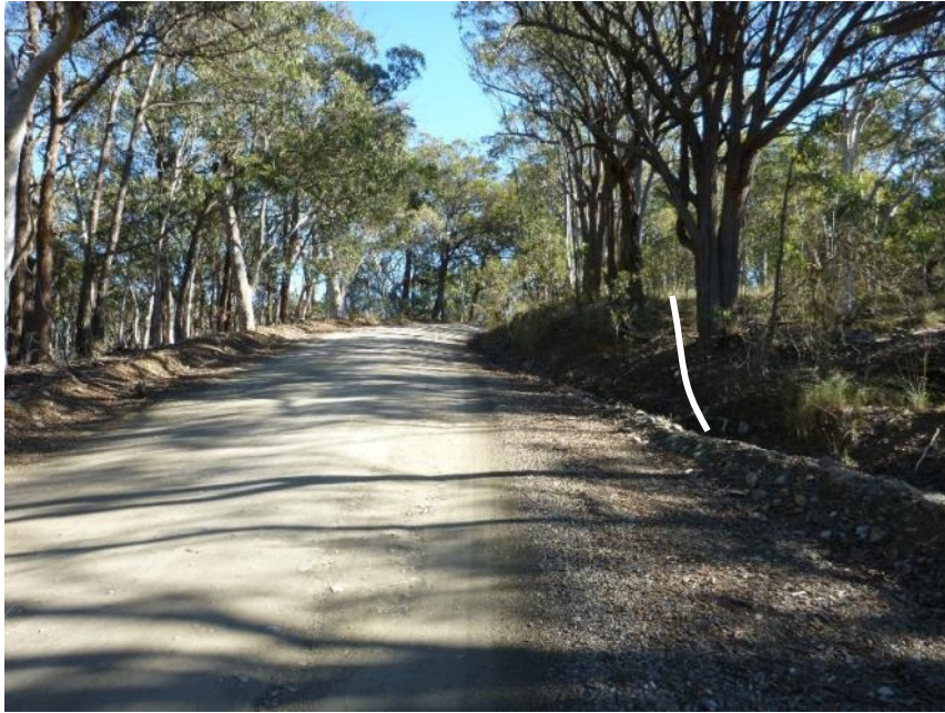
Plate 43 Location of Upgrade 3.23 ; looking 230°.
