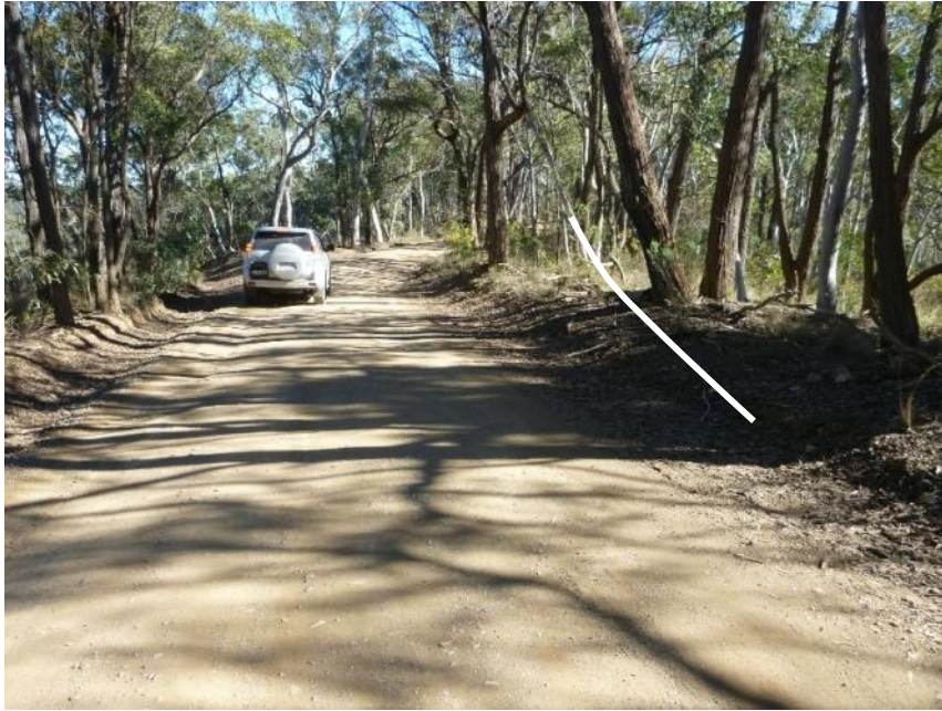
Plate 37 Location of Upgrade 3.20 ; looking 230°.
