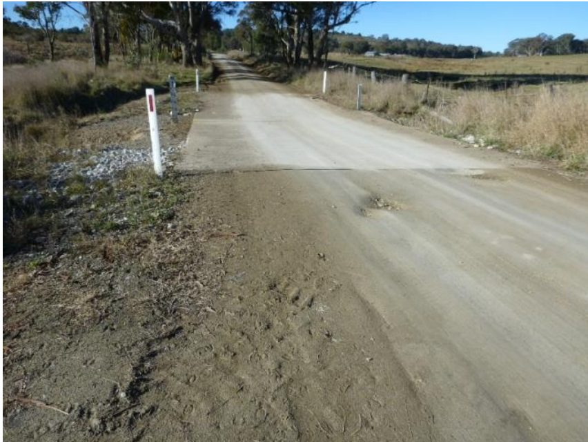
Plate 58 Location of Upgrade 3.29 ; looking 50°.
