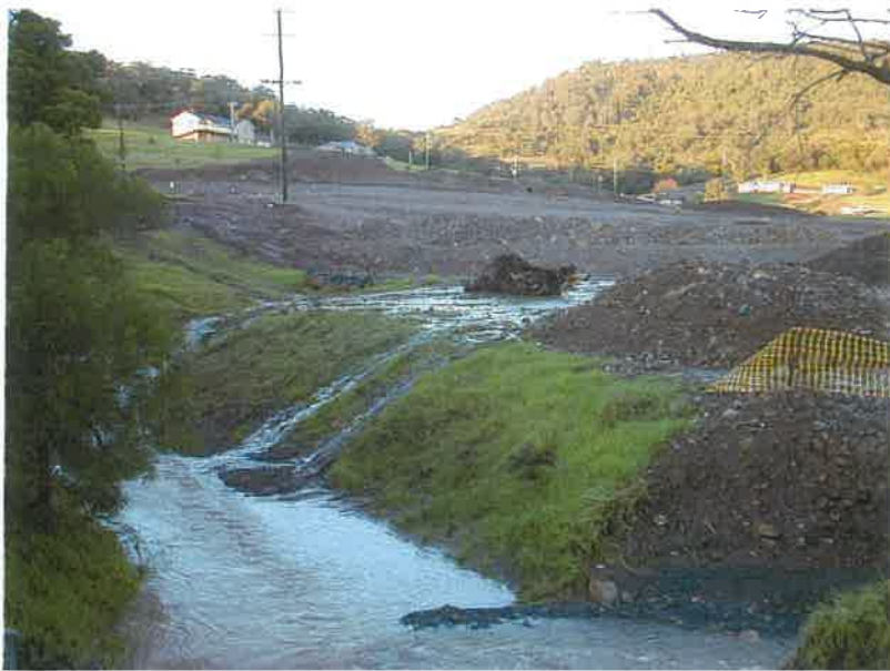
Figure 8 Highly turbid stormwater discharging from a housing development under construction at Albion Park.
