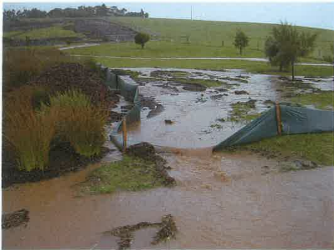
Figure 3 Sediment controls associated with a housing subdivision under construction being overwhelmed during a rainfall event (Elambra Estate near Gerringong).
