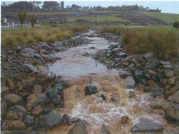
Figure 4 Highly turbid stormwater emanating from a housing subdivision under construction during a rainfall event (Elambra Estate near Gerringong).
