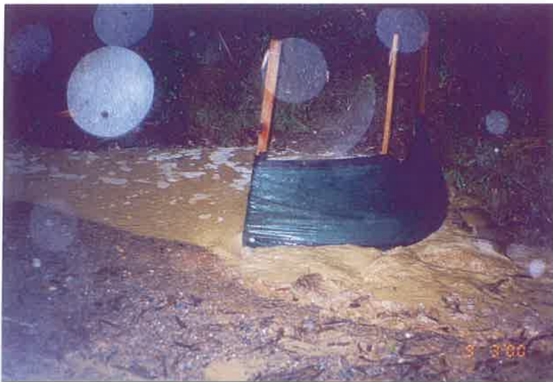
Figure 10 Highly turbid stormwater from a housing development under construction overwhelming a sediment fence.
