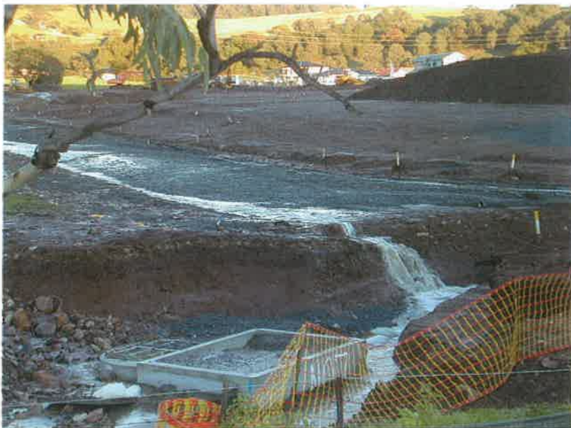
Figure 9 Highly turbid stormwater discharging from a housing development under construction at Albion Park.
