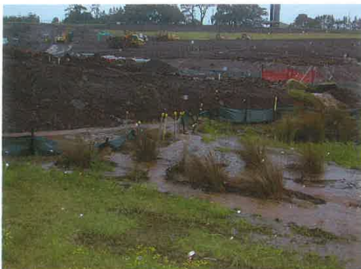
Figure 5 Sediment controls associated with a housing subdivision under construction being overwhelmed during a rainfall event (Elambra Estate near Gerringong).
