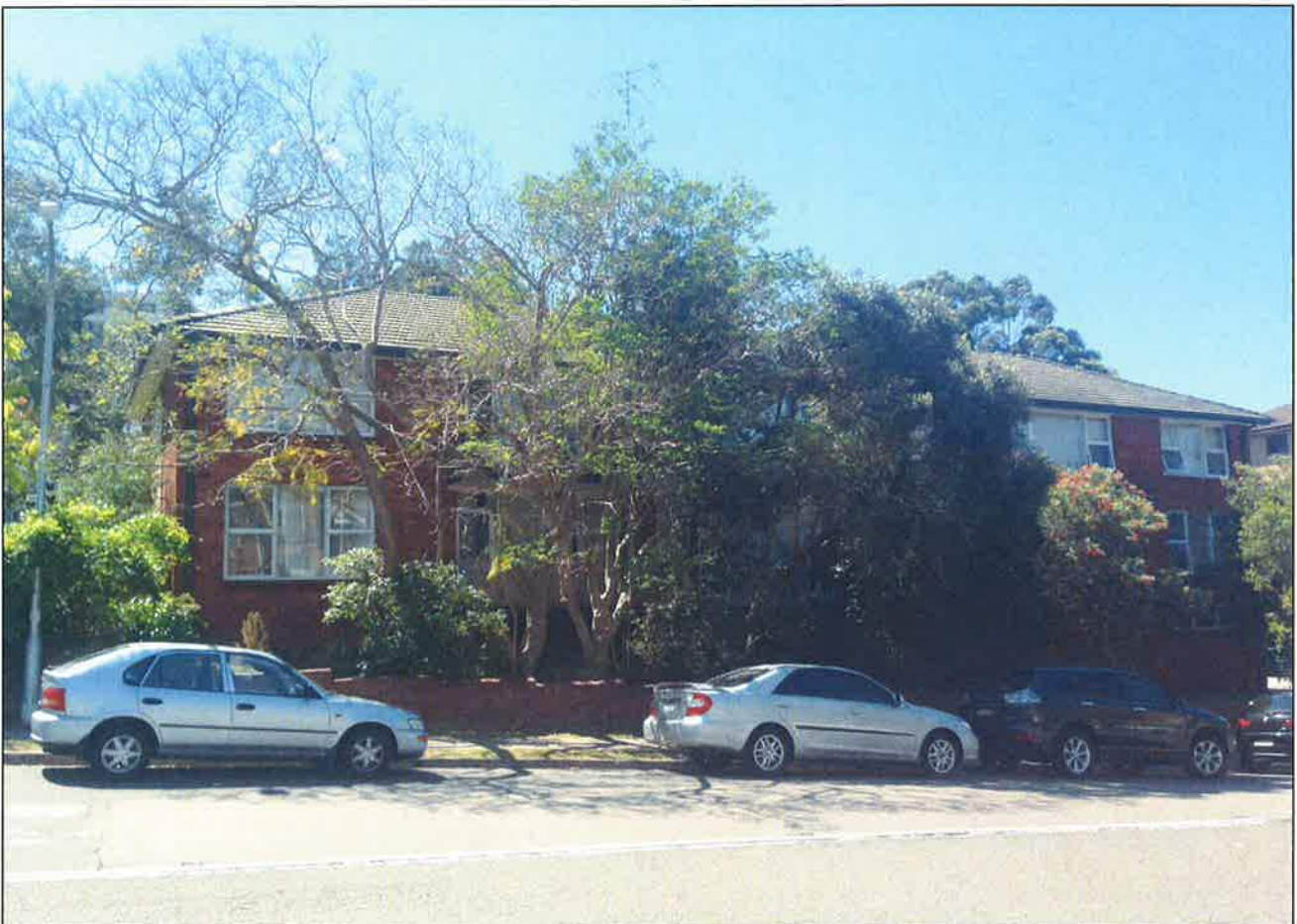
Figure 12: Western façade of 522 Railway Parade showing dense tree planting
