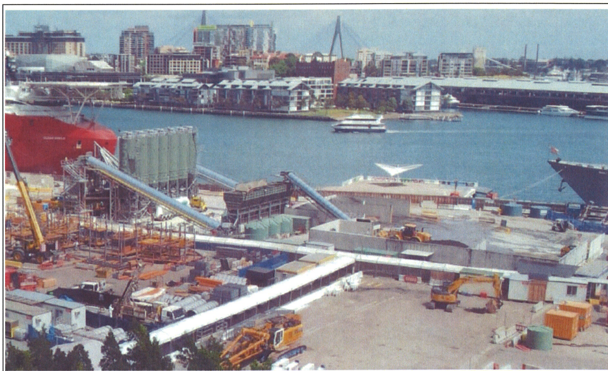
Figure 4: View of the temporary concrete batching plant looking west across Barangaroo South
