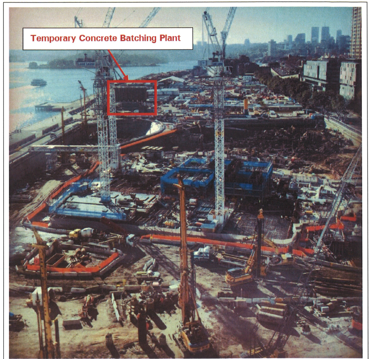
Figure 5: View of the temporary concrete batching plant looking north across Barangaroo South.
