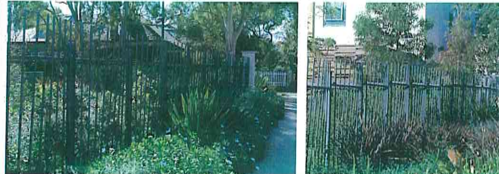
PALISADE STEEL FENCES
