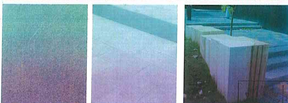
EXPOSED AGGREGATE CONCRETE PAVING
