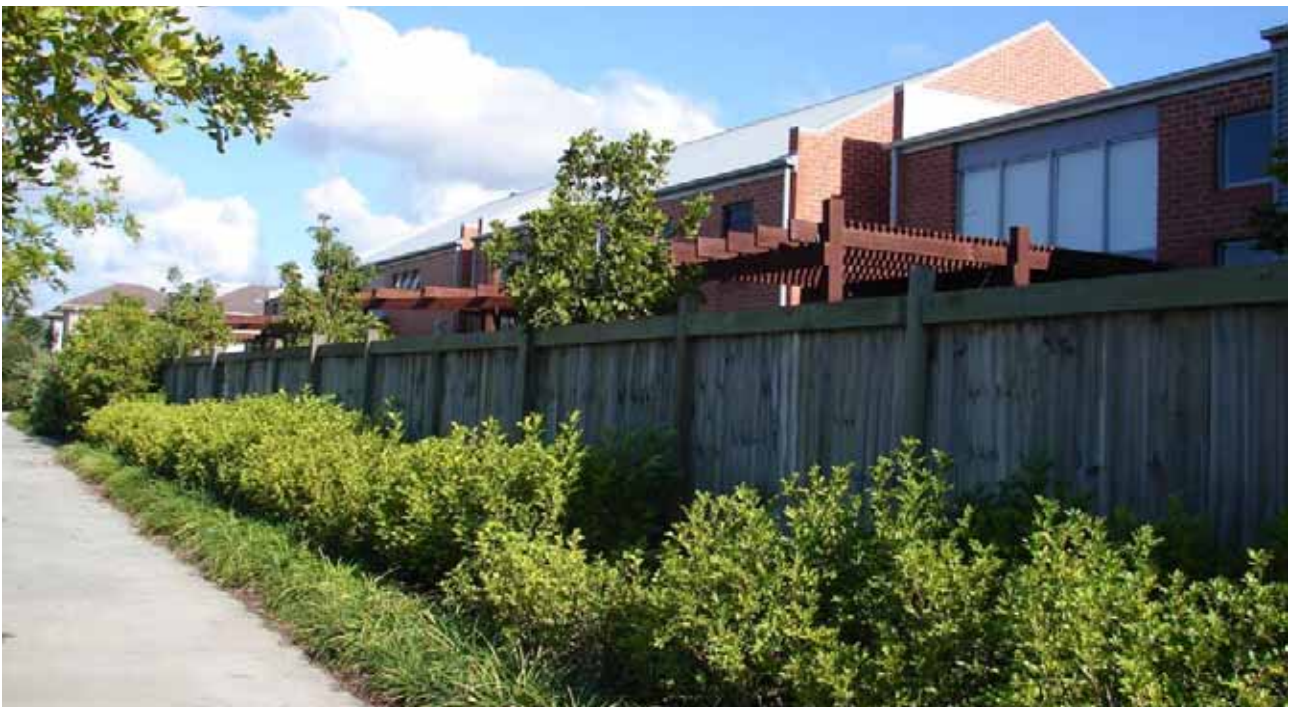
Single Frontage Terrace Dwelling with Double Garage at Varsity Lakes (back view)
