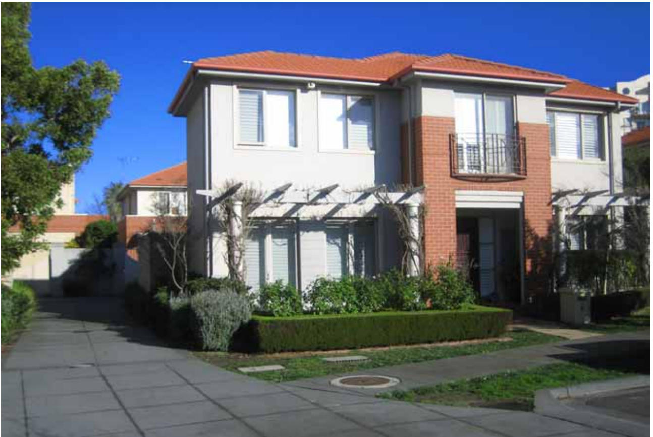
Mews Product Containing Four Dwellings Accessed via a Shared Central Driveway
