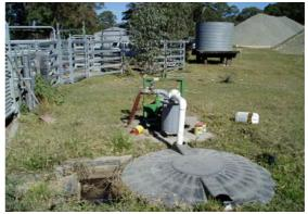
**Plate 1:** Spray race pump, sump and underground water supply/mix tank.
