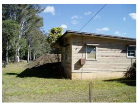
**Plate 12:** View to front of on-site house showing painted wood with significant flaking of paint.
