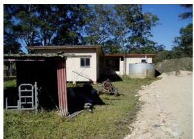
**Plate 11:** View to rear of on-site house showing fibro sheeting used as external cladding.
