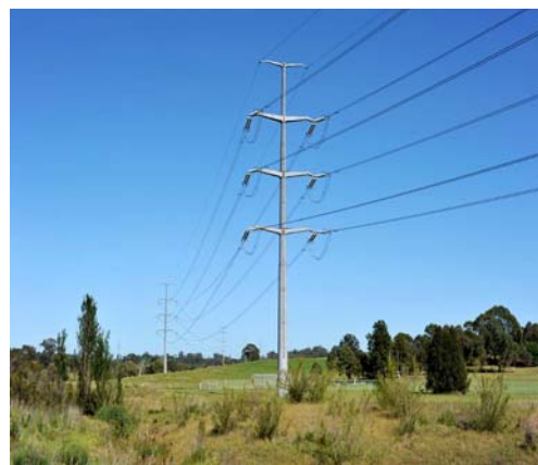
Plate 12 – Typical illustration of a 330 kV supporting structure
