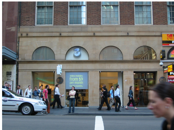
Figure 3-5 The ground floor façade was modified a number of times since the 1960s, when the original shop front was removed and replaced with sandstone arcade. Components of the original fabric including the awning and characteristic Georgian type glazing bars of the semi-circular fanlights have also been lost.
