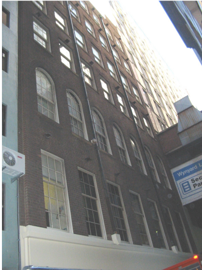
Figure 3-3 The rear façade retains its face brick upper section and multi-paned timber windows.
