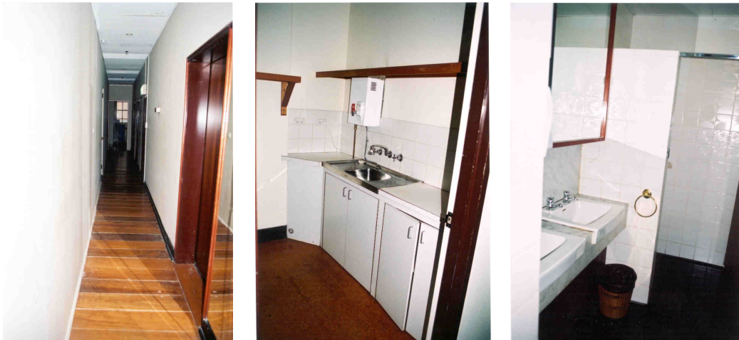
Figure 3-25 The exposed timber floor at third level may be part of the original 1923 fabric of the building. Kitchen and toilet fitouts date from 1971 or more recent alterations throughout the building.
