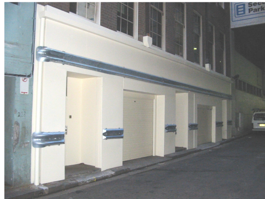
Figure 3-7 The stone base of the rear façade has been altered, covered with metal plates for protection and painted over. A new rear entrance was formed in 1971, one loading dock created in 1995 and another in 2003.
