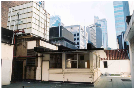
Figure 3-10 Looking east on the roof. Note 1971 store structure, which was built on the top of the former light area. The tiled roof in the background is part of the original design. The timber wall is later addition.
