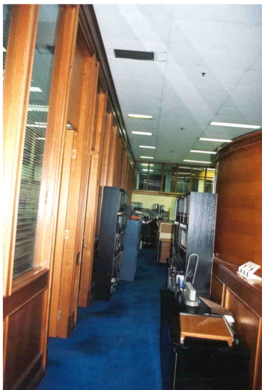
Figure 3-19 The fitout of first floor office space appear to date from the 1971 major refurbishment. Note full-height timber and glass partitions and false ceiling
