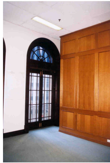
Figure 3-22 Office space facing George Street. Note original timber door with semi-circular fanlight
