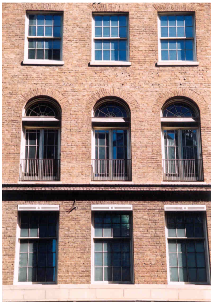
Figure 3-4 Detail of the upper section of the façade featuring excellent materials and detailing. Note multi-paned timber framed windows and semi-circular fanlights to second floor windows.
