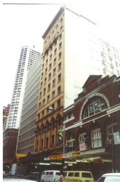
Figure 4.5 Masonic Club, 169-173 Castlereagh Street, Sydney. Architect: C. W. Chambers Construction: Reinforced Concrete frame, sandstone exterior with trachyte cladding to street. Inter War commercial palazzo, 1925 (source: Brian McDonald & Associates 1996)
