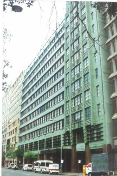
Figure 4.7 Transport House, 11-31 York Street, Sydney Architect: H.E. Budden & Mackay Construction: 1934-36 Inter War Art Deco. – Façade clad with - Glazed terracotta tiles (source-Brian McDonald & Associates 1996)
