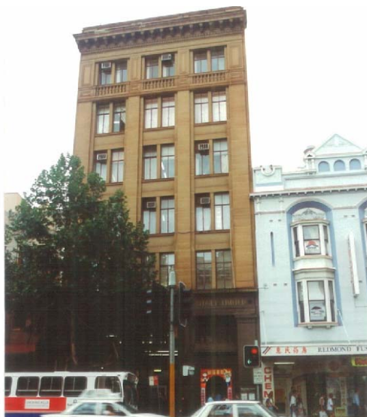
Figure 4.4 National Australia Bank, 661-663 George Street, Sydney. Architect: Kent & Massie Construction: Reinforced Concrete frame, sandstone and granite exterior Inter War commercial palazzo, 1925 (source: Brian McDonald & Associates 1996)
