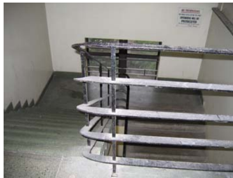
Photograph 3.7: illustrates typical metal balustrade to fire stair. (source: Photograph taken by Brian McDonald of HBO+EMTB Heritage Pty Ltd, February 2005)
