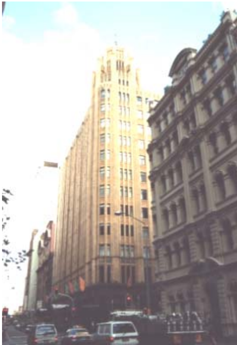
Figure 4.6: Grace Building, 77-79 York Street, Sydney Architect: Morrow and Gordon Construction: 1928-10 Inter War Skyscraper Gothic Art Deco detail. – Façade clad with - glazed terracotta tiles (source-D. McBeath 1997)
