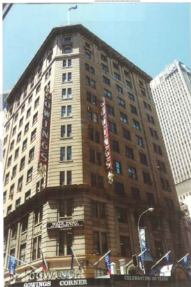
Figure 4.3 Gowings Department Store, 452-456 George Street, Sydney. Architect: Robertson & Marks Construction: Reinforced Concrete frame, sandstone exterior Inter War commercial palazzo, 1912-1929 (source: Brian McDonald & Associates 1996)
