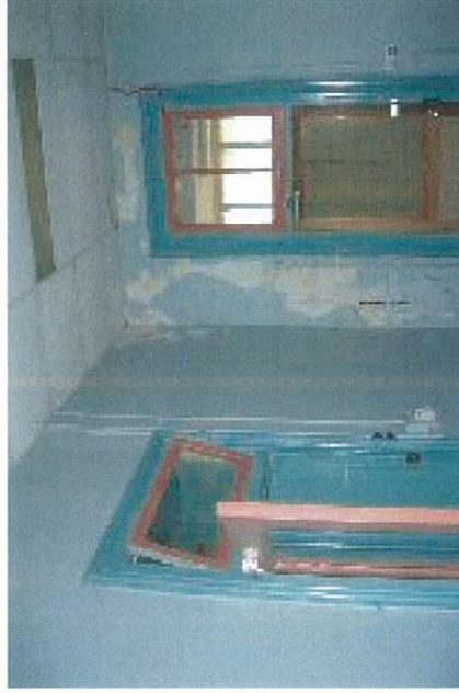
Chief Mechanical Engineer's Building - Interior
