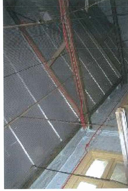
Telecommunications Building - Interior
