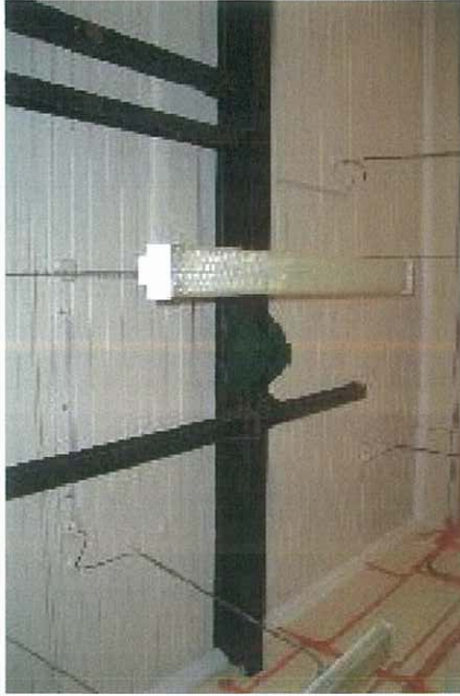
Scientific Services Building - Interior
