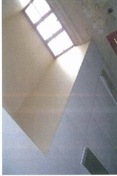
Chief Mechanical Engineer's Building - Interior
