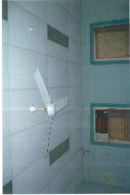
Chief Mechanical Engineer's Building - Interior
