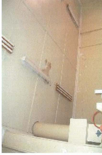
Scientific Services Building - Interior
