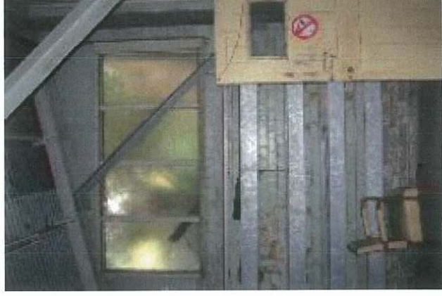
Telecommunications Building - Interior
