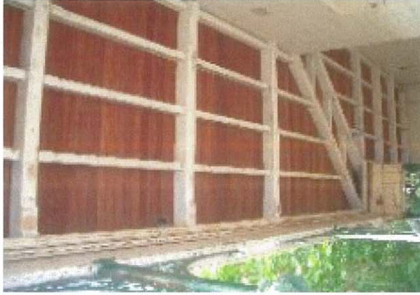
Chief Mechanical Engineer's Building - Exterior
