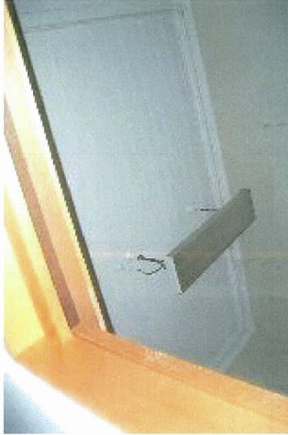
Chief Mechanical Engineer's Building - Interior
