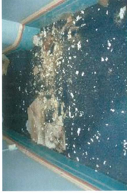
Chief Mechanical Engineer's Building - Interior
