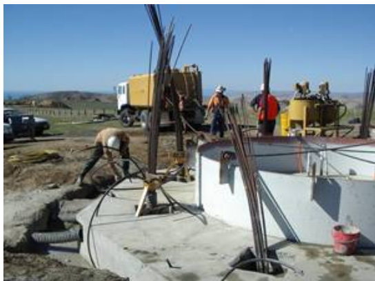
Plate 4-1: Foundation pad construction components
