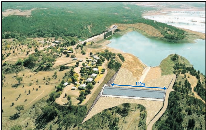
Option D3 - Spillway alternative. Saddle dam alternative 2.3m higher than Option B1
