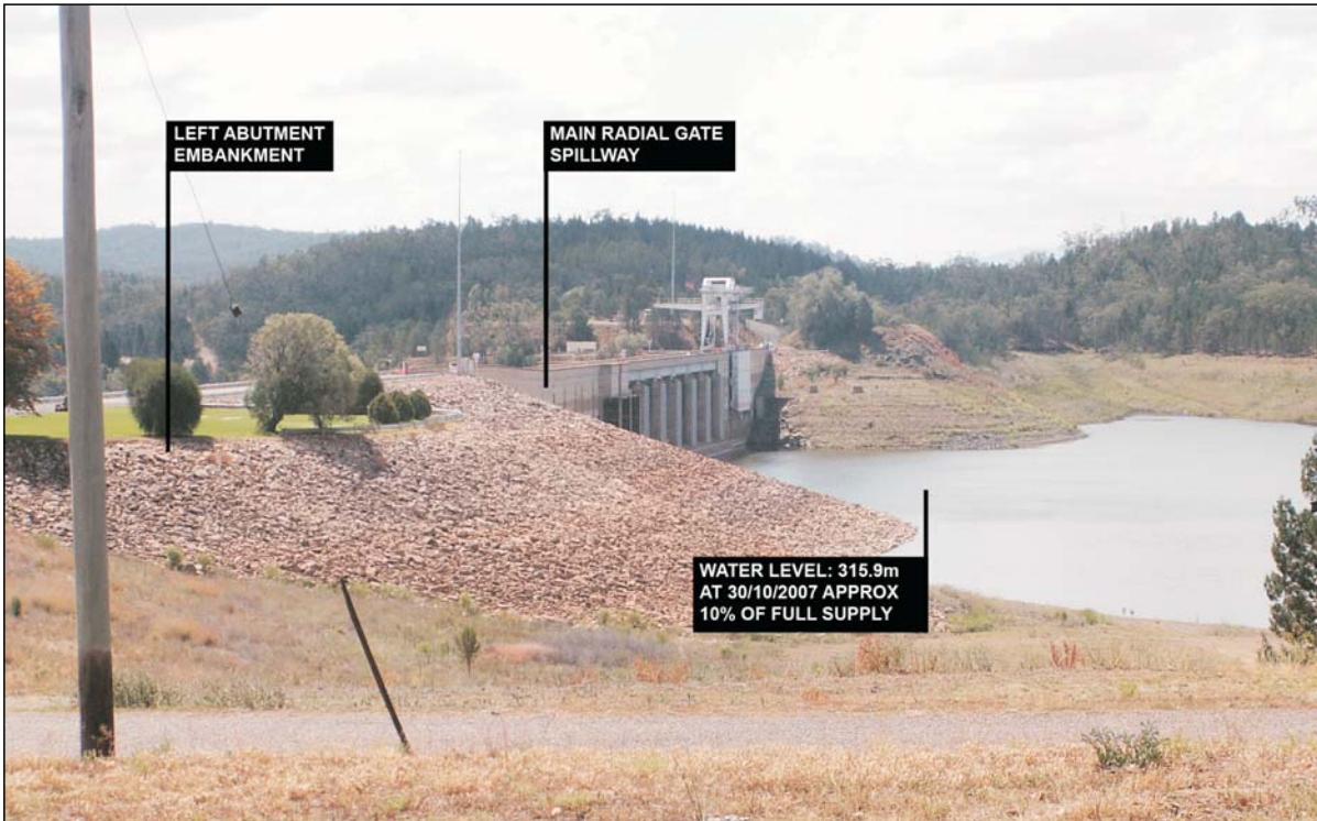
Existing - Looking north west to main spillway from VP7
