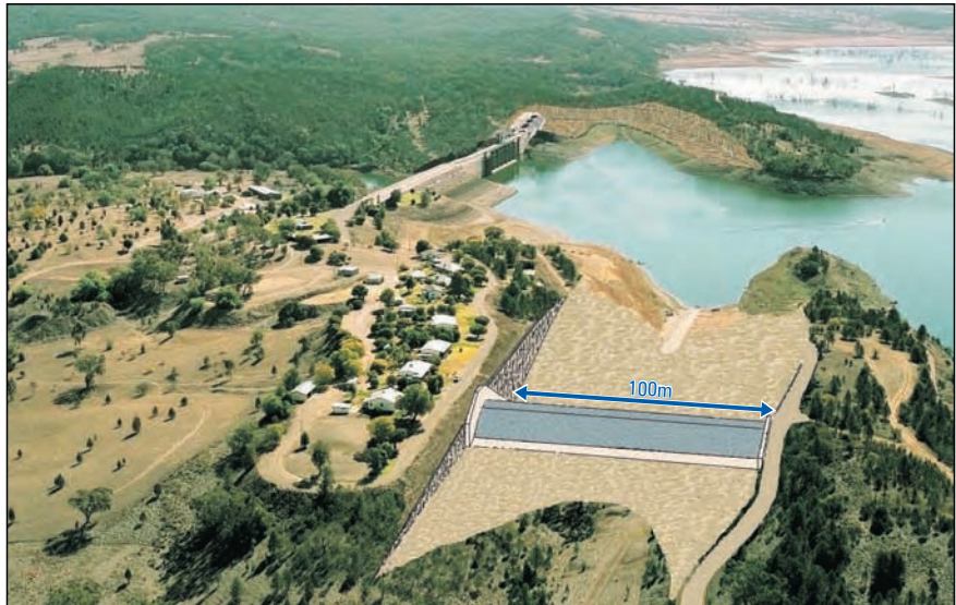
Option D2 - Spillway alternative. Saddle dam alternative 1.4m higher than Option B1
