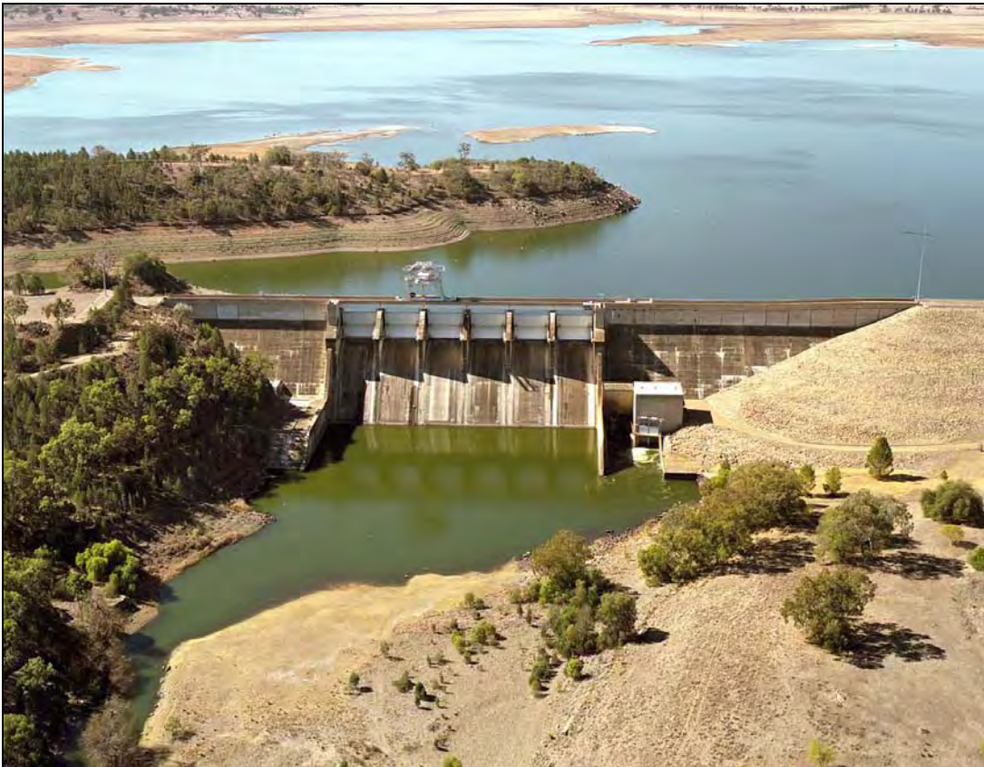
Photograph 1.1 The existing main dam wall
