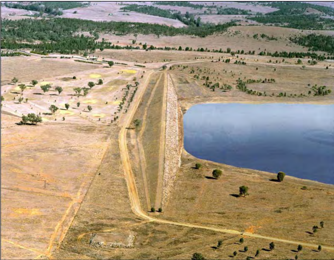
Photograph 1.2 The existing subsidiary dam wall
