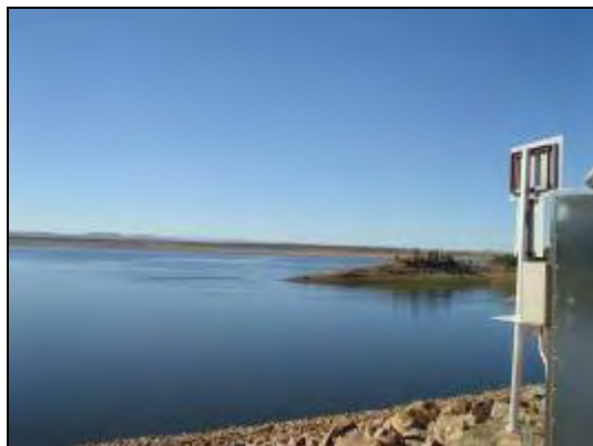
Figure 24 View of water storage area from spillway (facing east).
