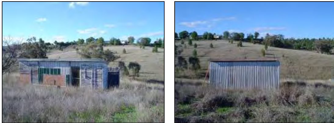
Figure 21 Views of the School/Scout Hall complex.
