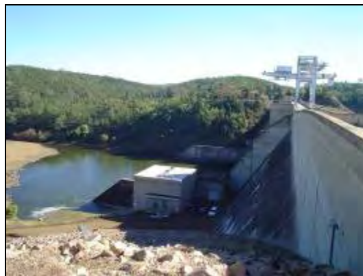
Figure 25 View of spillway (facing northwest).
