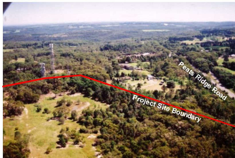
Plate 4.7: Oblique aerial view to the west across the vegetation screen along the western boundary of the Project Site (Ref: 521E/29)
