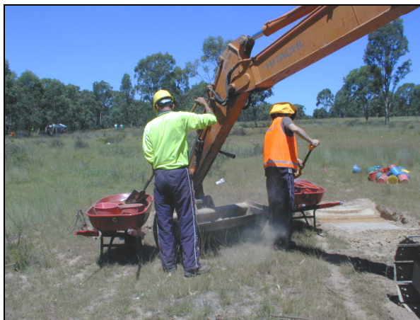
Plate 6.3 Removing deposit from backhoe bucket
