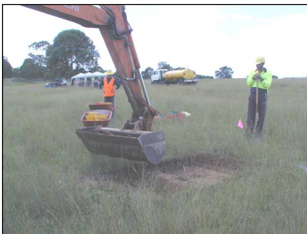
Plate 6.1 Initial grass and topsoil removal
