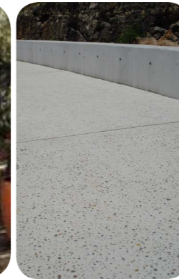
In situ concrete footpath with exposed aggregate > ASPECT image library
