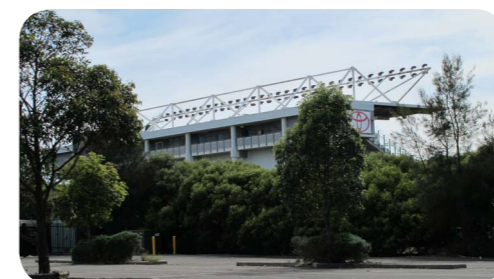
Carpark on western side of stadium
