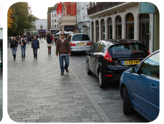
Flush kerbs and parking bays
