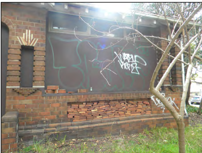
Figure 27: Detail of the northern side of the front elevation. The brickwork is in poor condition.
