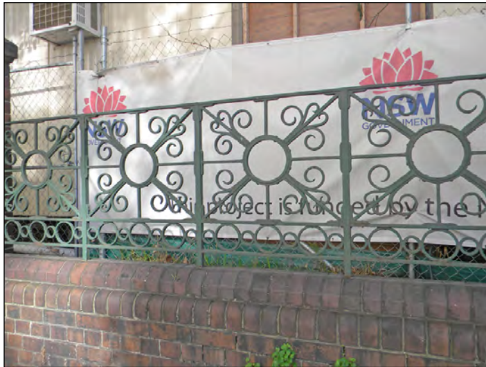
Figure 41: Detail of the wrought iron panels in the front fence.
