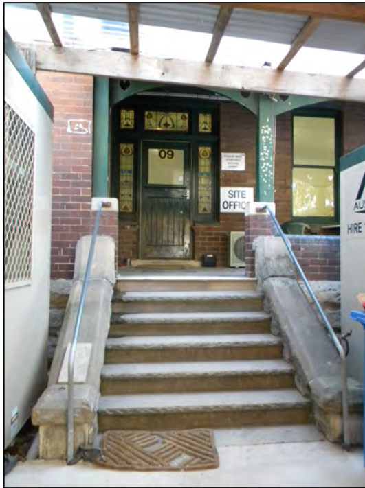
Figure 45: Detail of the stone capped stairs leading up to the verandah and of the front door.
