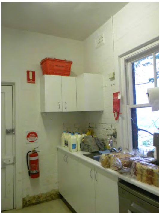
Figure 82: Painted brick walls, square set ceiling and kitchen fit out in Area 13.
