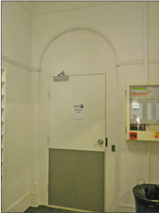
Figure 58: Fire door separating Areas 1 and 2. Note the arch in the wall.
