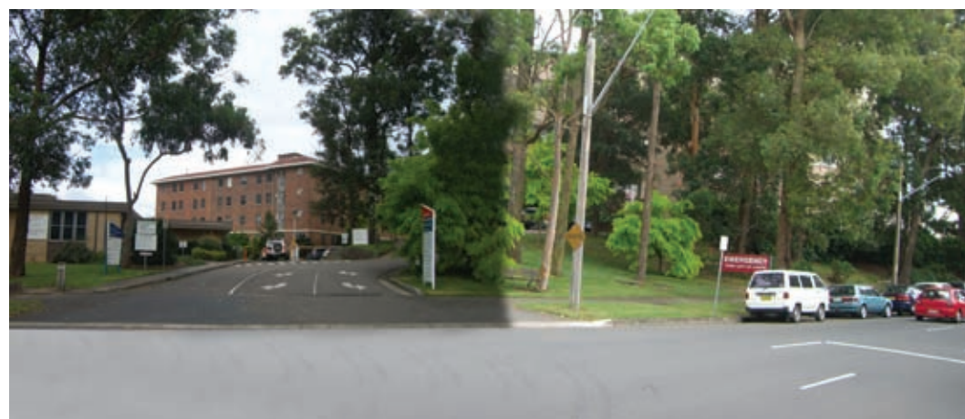
The Emergency entrance off Fox Valley Rd
