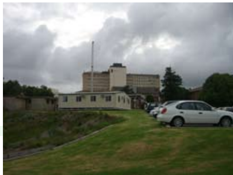
Looking towards the main hospital building from Southern part of site
