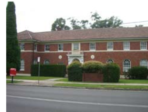
Existing heritage Administration building
