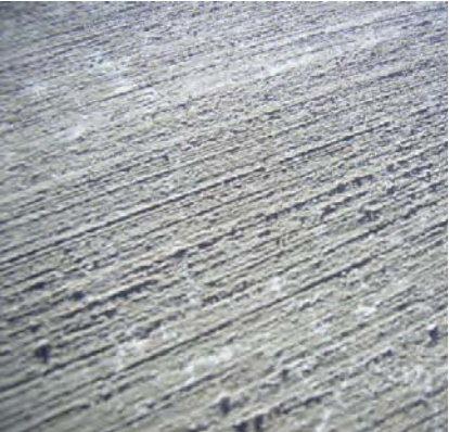
Above: Broom Finish Concrete
