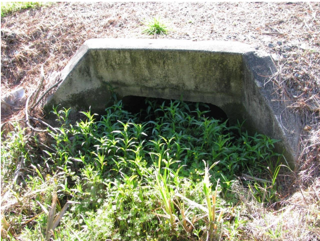
Photograph 2 – Small existing culvert will be retained to drain the existing table drain
