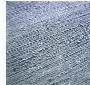
Above: Broom Finish Concrete
