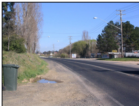
Photograph 14: The Great Western Highway west of the existing access
