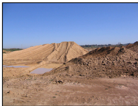
Photograph 4: Stock piling on site
