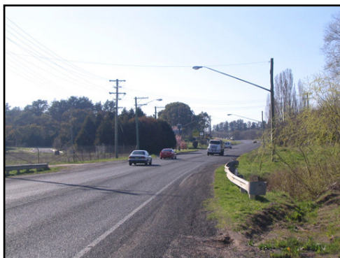
Photograph 13: The Great Western Highway east of the existing access
