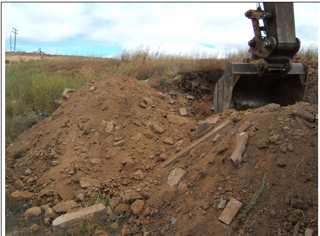
Figure 5 Test Pit 1 – Concrete and brick rubble underlain by fuel-stained soil
