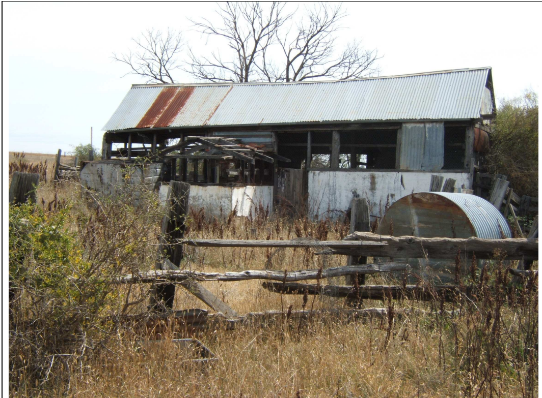
Figure 3 Former Ingersole's Abattoir (circa 1910) view from south
