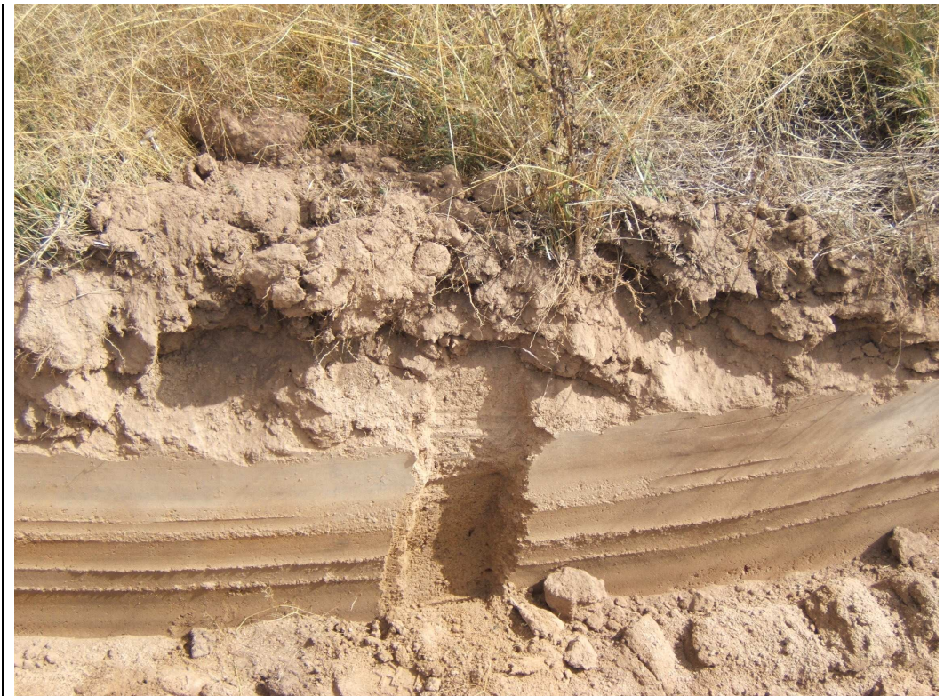
Figure 4 Test pit from east side of the central Unnamed Creek upslope showing shallow sandy profile above weathered granite (Test pit 20)
