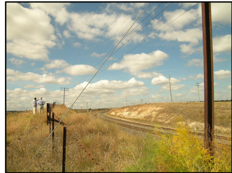
Photograph 8: Existing rail line looking west
