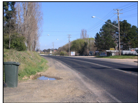
Photograph 4: Great Western Highway looking west
