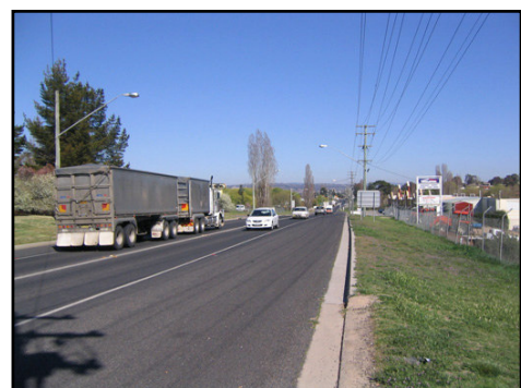
Photograph 6: Typical heavy and light traffic at Great Western Highway
