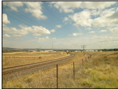
Photograph 7: Existing rail line looking east
