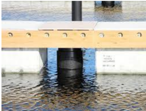
Figure 2 Telescopic Pile
