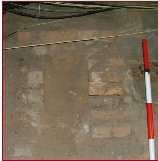
Figure 29. View of sandstock brick box drain, visible in section. (AHMS 2007b)
