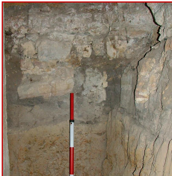
Figure 28. View of sandstone footing visible in section (Source AHMS, 2007b)
