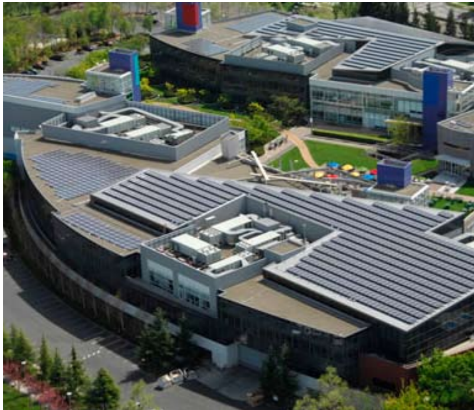
Figure B4.4.1 - Photovoltaic solar panels on roof of building
