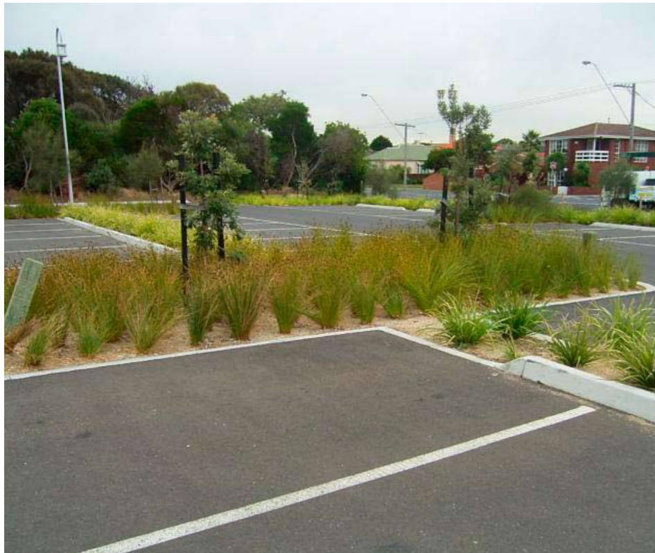
Figure B4.8.1 - Bioretention system in car parks
