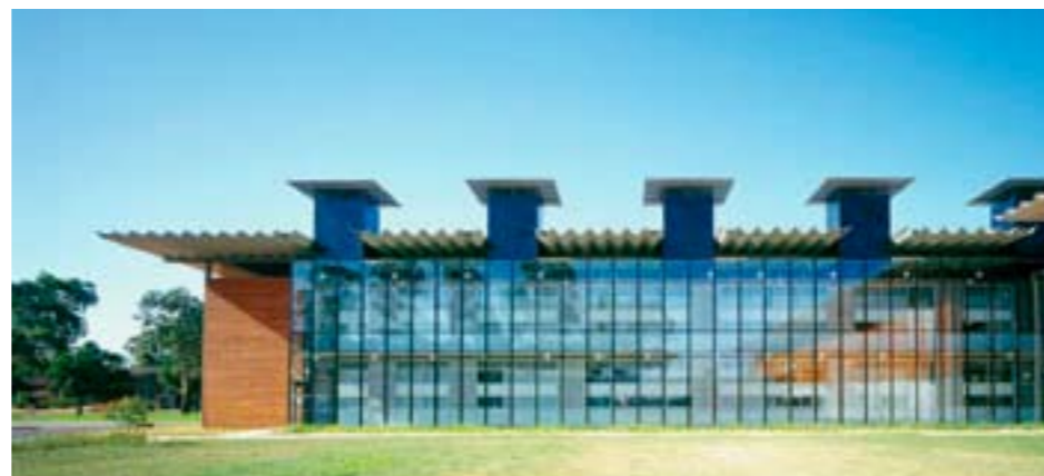
Figure B4.4.4 - Natural cross-ventilation or solar chimneys
