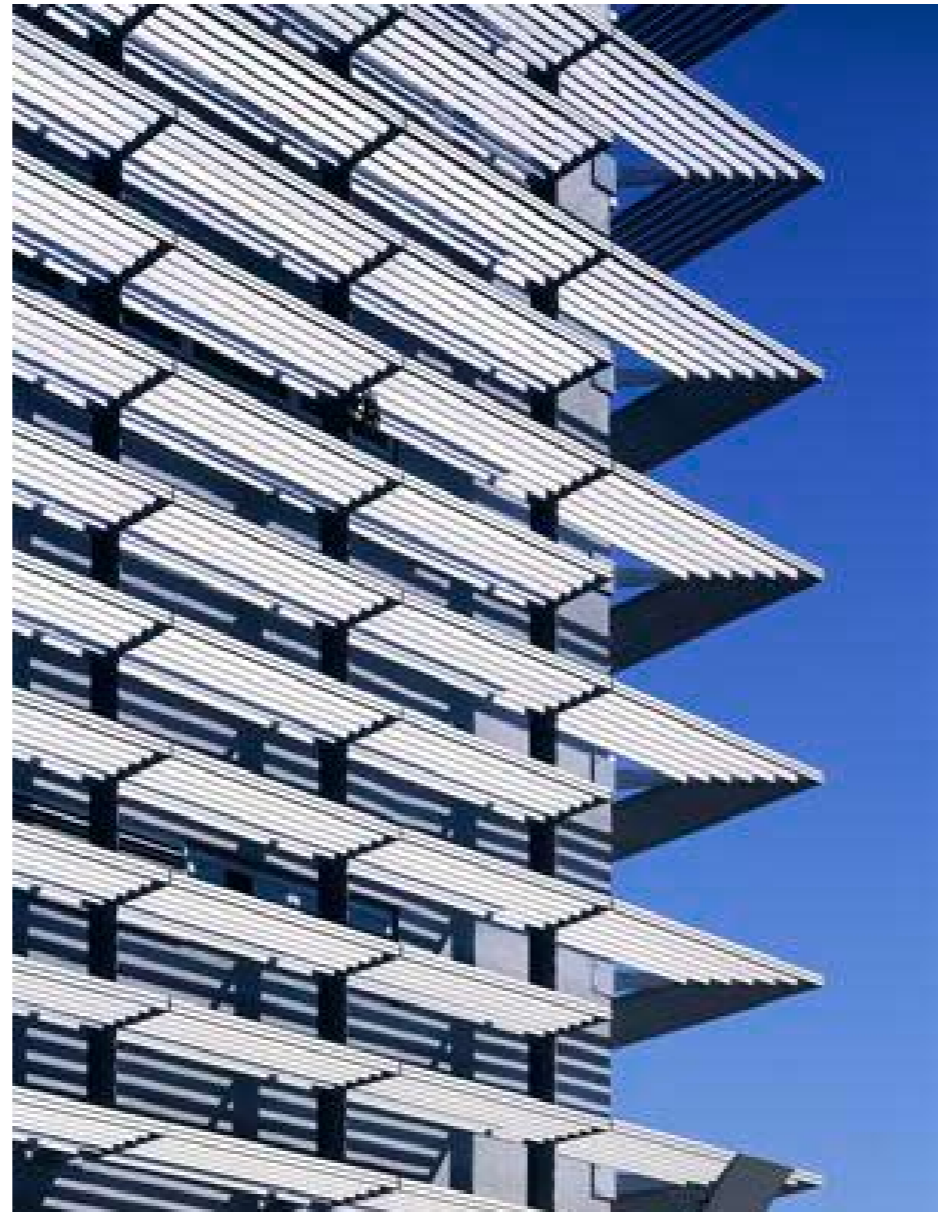
Figure B4.4.3 - Use of sunshading devices to enhance energy efficiency
