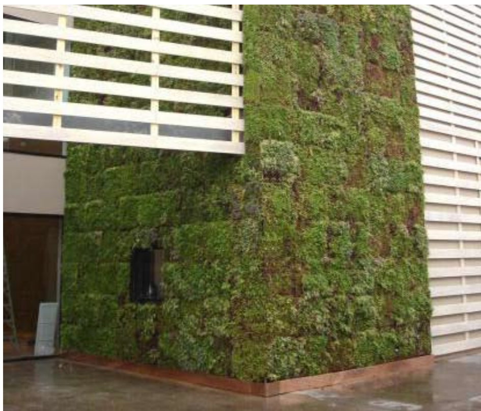
Figure B4.4.2 - Use of biowall to act as biofilter and enhance the aesthetic quality of the building
