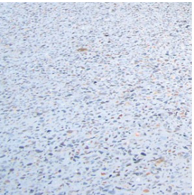
In-situ concrete pedestrian paths with exposed aggregate
