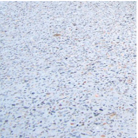
In-situ concrete pedestrian paths with exposed aggregate
