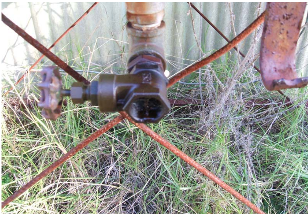
Photo 6: leaking heating oil
