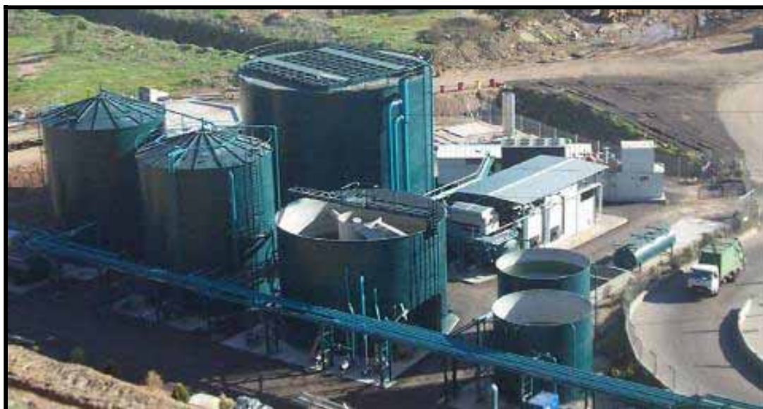
Figure 3.7: AWT Bioreactors Controlling Fermentation.
