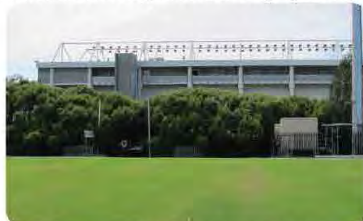
Western playing fields and drainage channel
