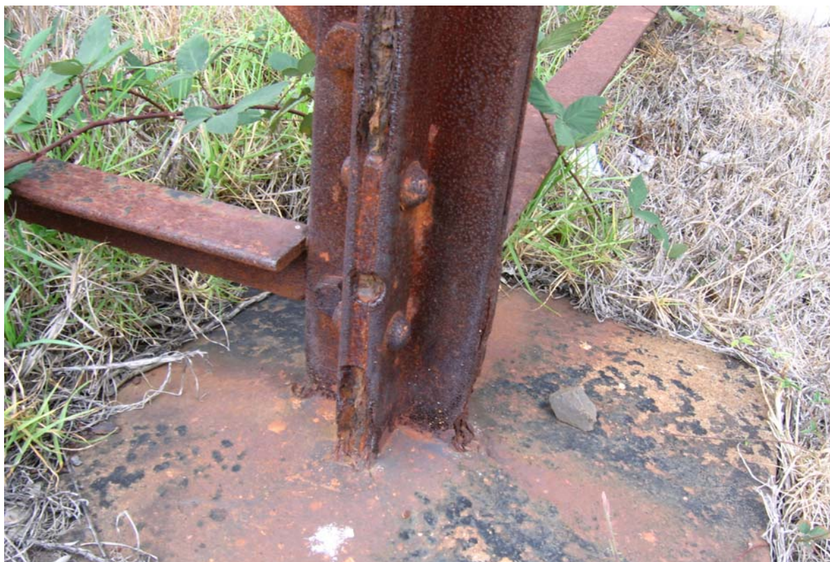
Photograph 9: Severely corroded steel at base of 1909 bridge support.
