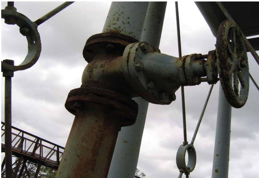
Photograph 4: Valve to inlet pipe under tank.
