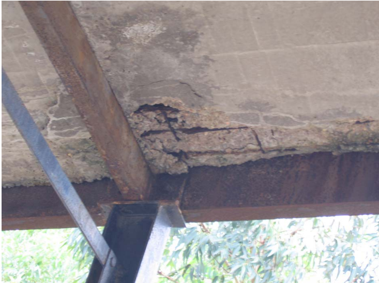
Photograph 15: Spalling concrete at underside of ramp.
