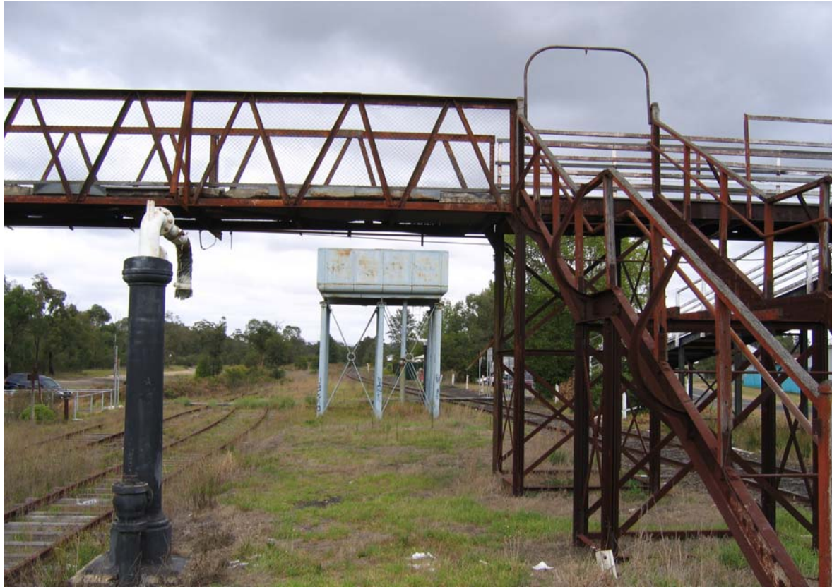
Photograph 10: Later phase trussed girder bridge abutting 1909 bridge and stair.
