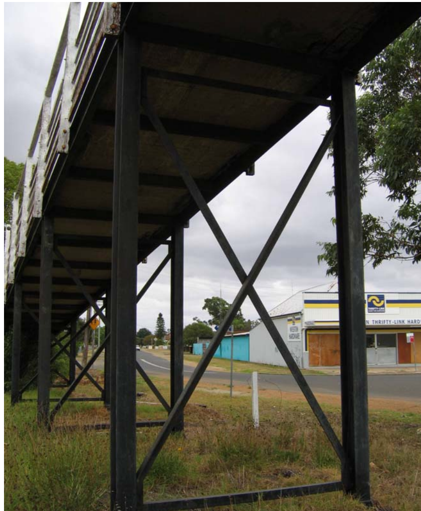
Photograph 14: Underside of northern ramp and support trestles.
