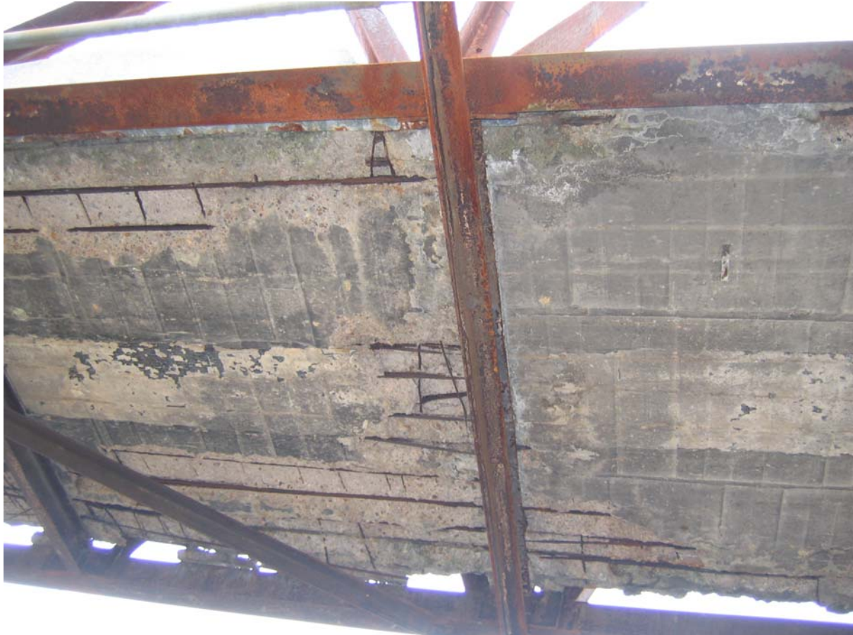
Photograph 12: later phase bridge. Severe spalling to concrete deck due to corroded steel reinforcement.
