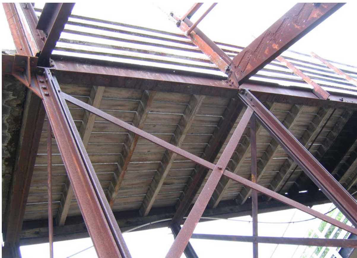
Photograph 8: Timber deck of 1909 section of bridge.
