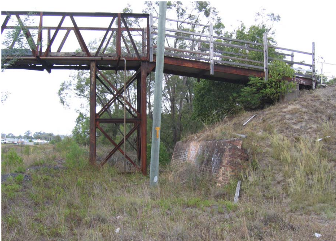
Photograph 11: Later phase bridge and support structure at brick abutment to southern ramped access.
