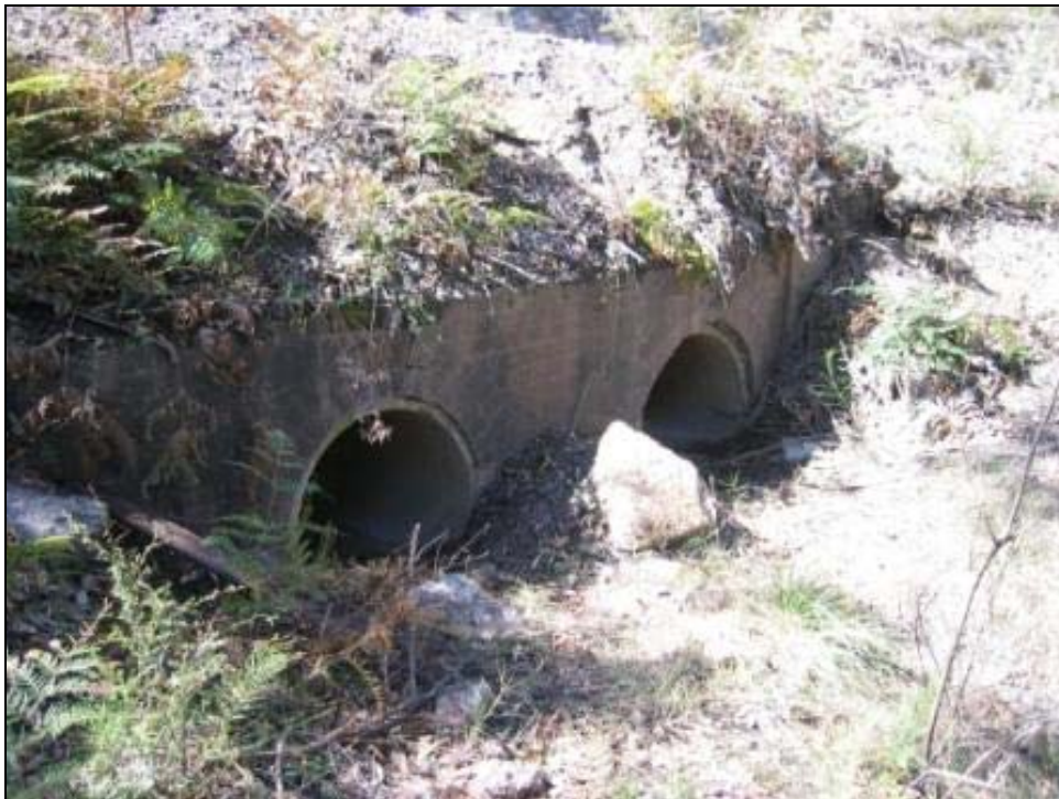
Plate 2 - Drainage culvert in buff coloured brick.
