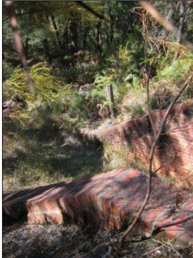
Plate 3 - Red brick abutment looking from rail bed.
