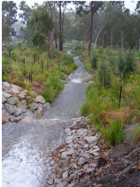
Figure 11 : Rock chutes under medium flow conditions at Lilac Street stream rehabilitation scheme
