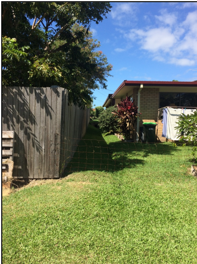
Photo 2: Swale drain at rear of existing properties.
