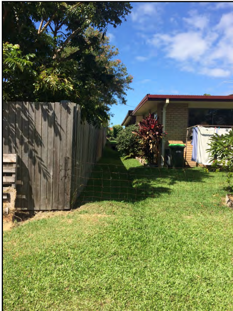
Photo 2: Swale drain at rear of existing properties.
