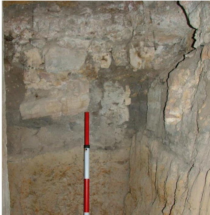
Figure 27. View of sandstone footing visible in section (Source AHMS: 2007b)
