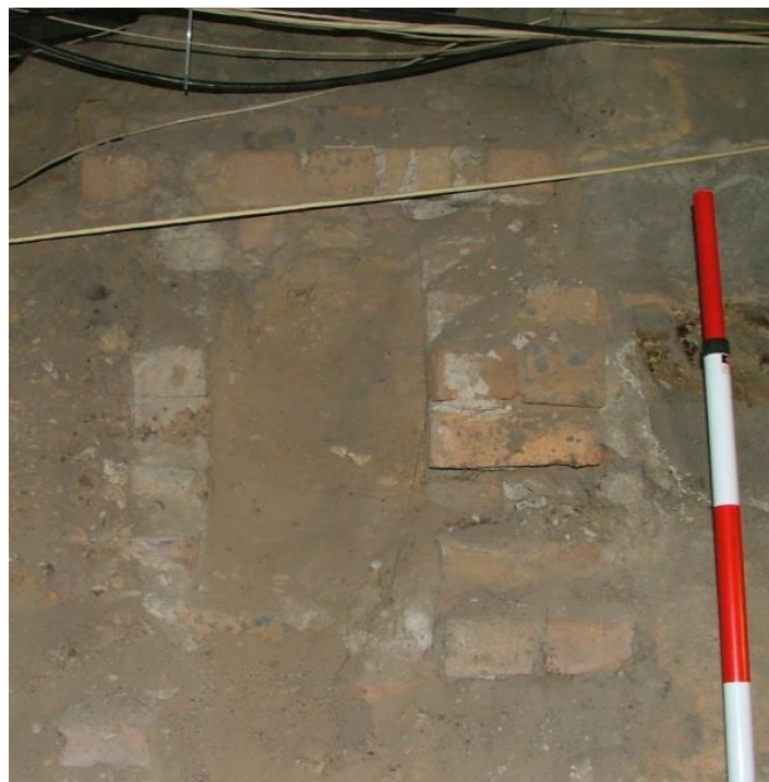
Figure 28. View of sandstock brick box drain, visible in section. (AHMS 2007b)
